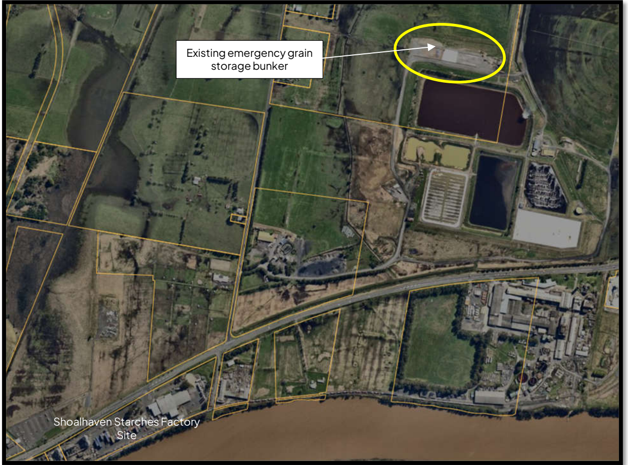
Figure 2: Aerial image of location of emergency grain storage bunker
