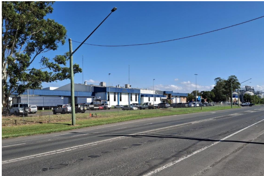
Plate 2: View of former Dairy Farmers factory and Shoalhaven Starches from Bolong Road frontage of subject land.
