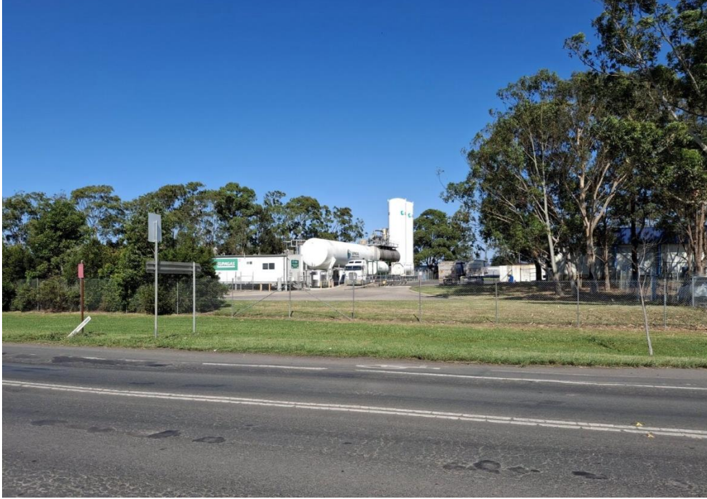
Figure 7 : View of the existing Supagas Plant. Proposed Storage vessels to be situated to rear of existing vessels visible in this view.
