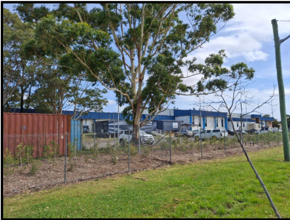
Figure 36: View of former Dairy Farmers factory building from Bolong Road.
