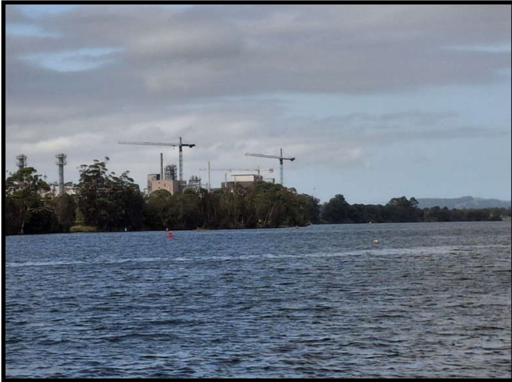
Figure 41: View of Shoalhaven Starches factory site from the vicinity of the Nowra Bridge over the Shoalhaven River.
