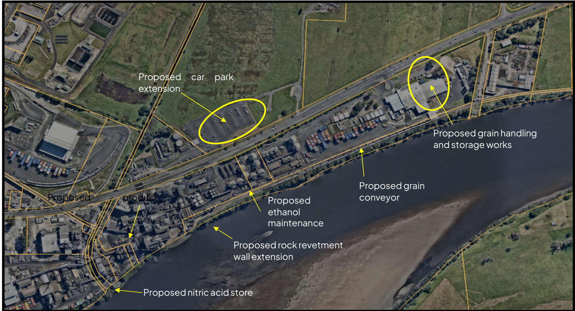
Figure 2: Aerial Image of location of proposed works within the Shoalhaven Starches factory site and former Dairy Farmers Factory Site
