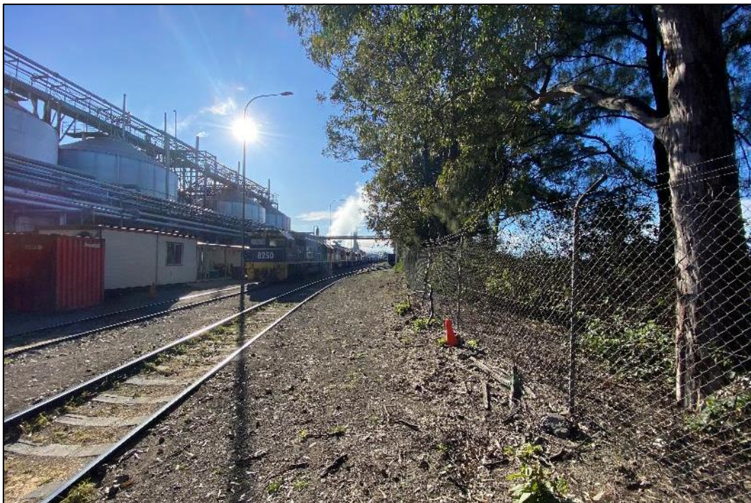
Plate 6: View along existing train line adjacent to the river bank.
