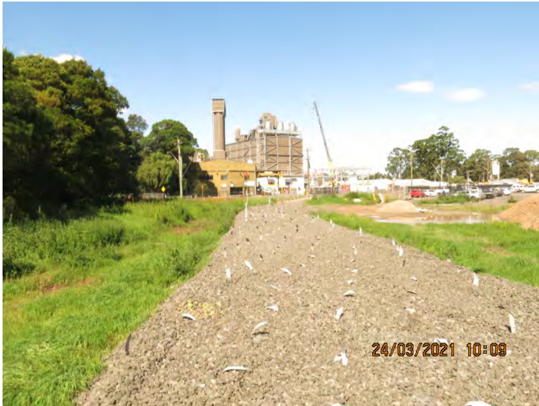
Photograph 9: Coarse gravel drainage layer in vicinity of perimeter road, with wick drains evident. Riparian corridor and Abernethy's Creek occur to east (left of photo). Note wick drains installed through drainage layer. The third rail siding will be positioned to west of the perimeter road (right side of photo).
