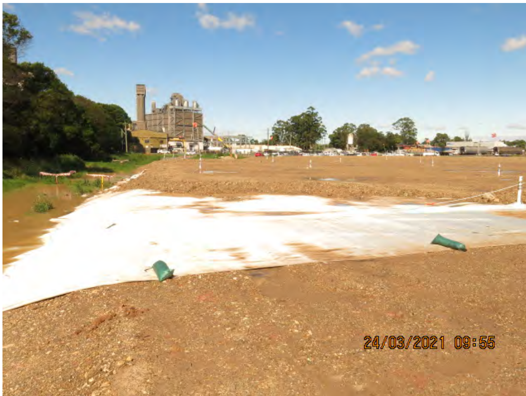
Photograph 8: View of site earthworks looking south, with structural geotextile exposed. Note settlement monitoring points and vibrating wire piezometer installations across the site. Note riparian corridor and Abernethy's Creek to east (left side of photo).
