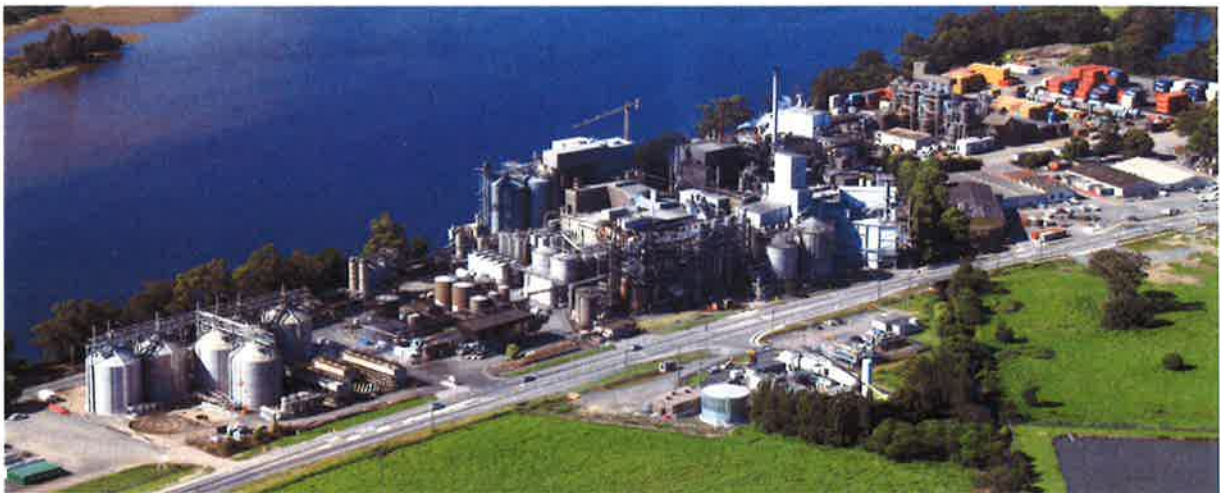
Shoalhaven Starches Factory, Bomaderry
