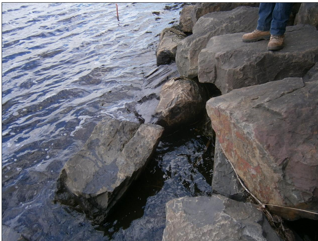
Photograph 5 – Displaced boulders at toe of rock revetment wall
