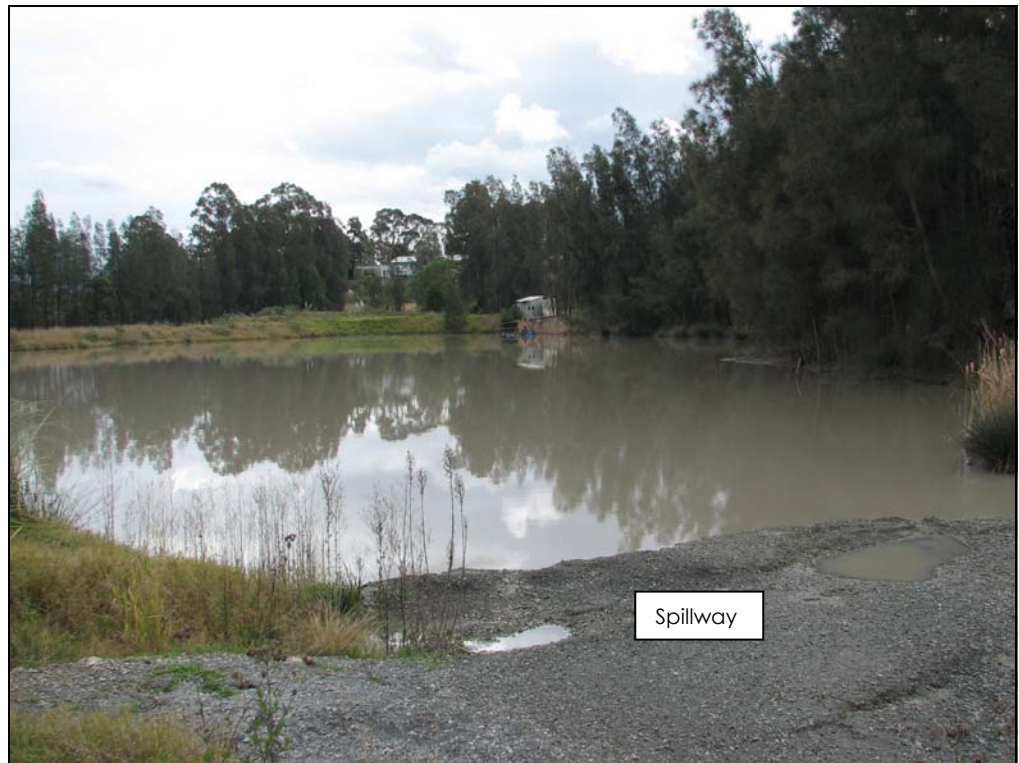
Plate 1: View to north west from spillway showing large sedimentation pond.
