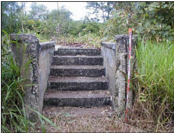
Plate 7.29 Concrete steps at KEH11
