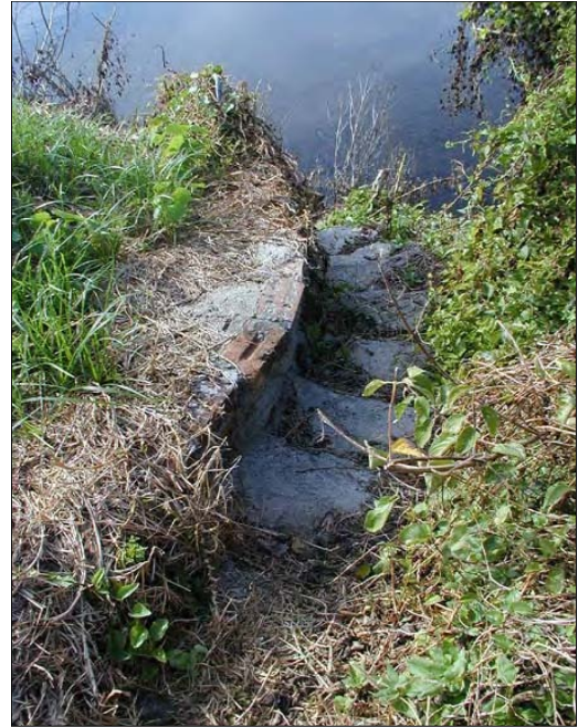
Plate 7.15 View of the concrete steps leading to a former wharf at the rear of the hotel
