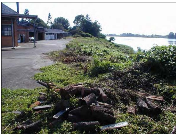
Plate 7.21 The rear platform behind the Butter Factory complex, looking northeast. A levee bank is proposed for construction between the bank and the structures.
