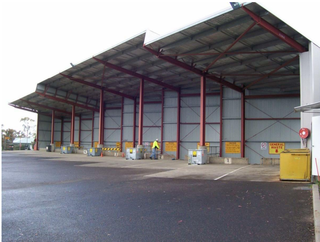
Plate 2: Armidale Waste Management Centre Disposal Bays
