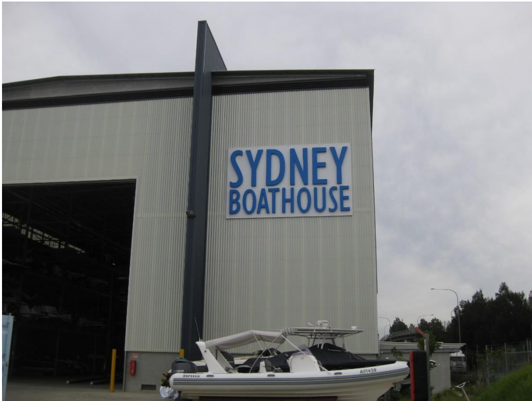
Figure 6: Existing business identification signage on eastern elevation of Western Boat Store
