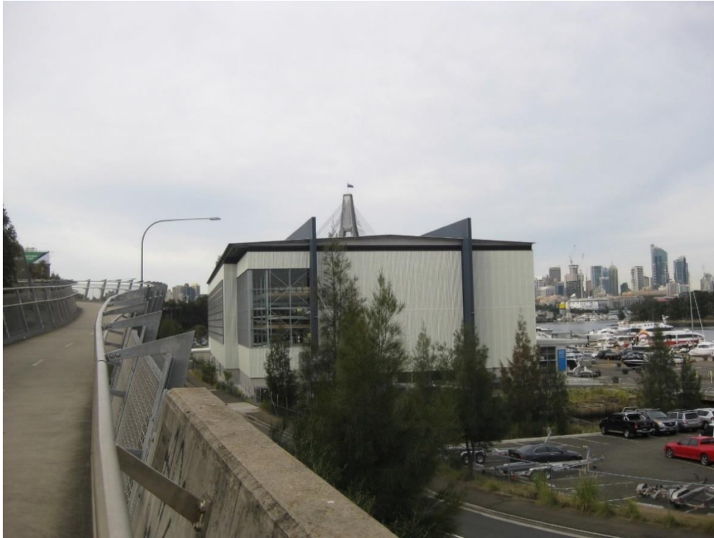
Figure 10: View from City West Link Pedestrian Overpass
