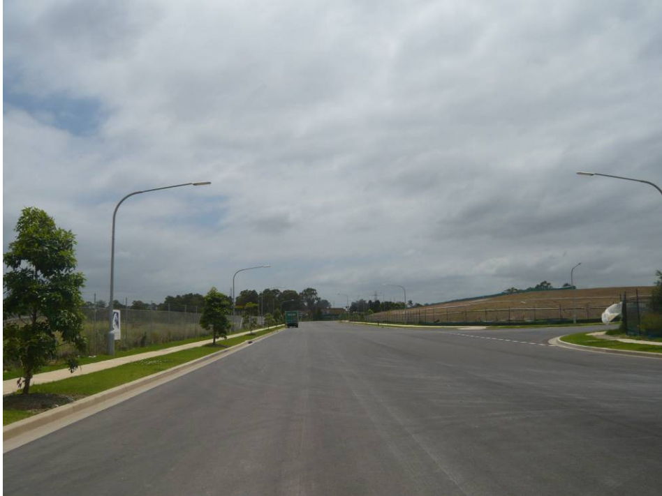
View looking north along Templar Road, towards its intersection with Lockwood Road
