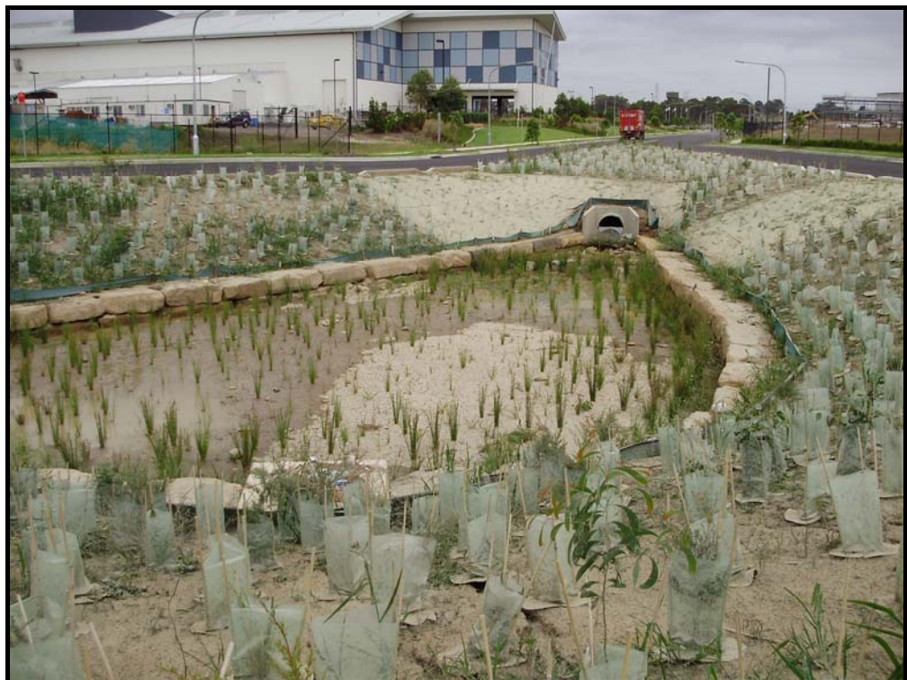
Photo 3 is a basin structure in the centre of a roundabout in Templar Road. The pipe outlet from this runs south, adjacent to the eastern boundary of Site H, then west adjacent to the southern boundary of Site H where flow discharges through a headwall shown in Photo 4.
