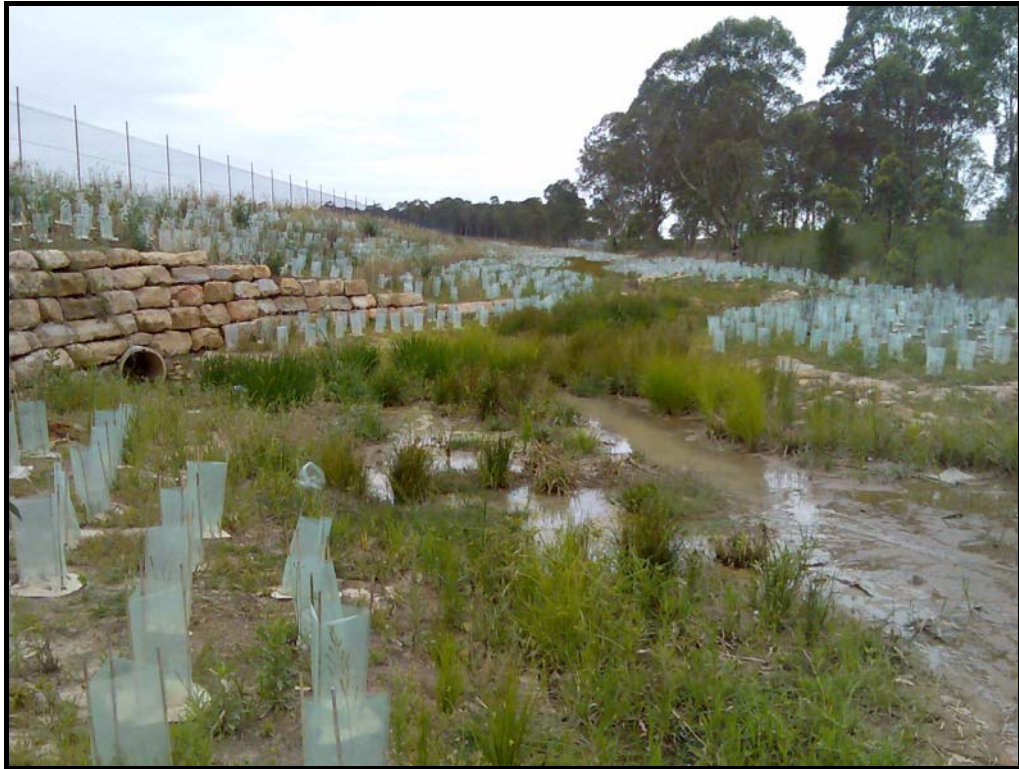
Photo 4 shows the headwall outlet as for the piped system described under Photo 3 and the drainage corridor which is generally wide with shallow banks on its south.
