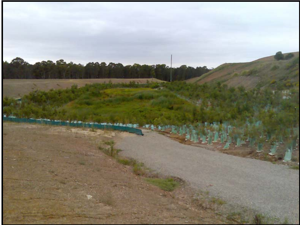
Photo 2 shows part of the existing Bluescope Steel stormwater detention basin that occupies a majority of the western boundary of Site H. This basin is proposed to be relocated to the south west corner of Site H
