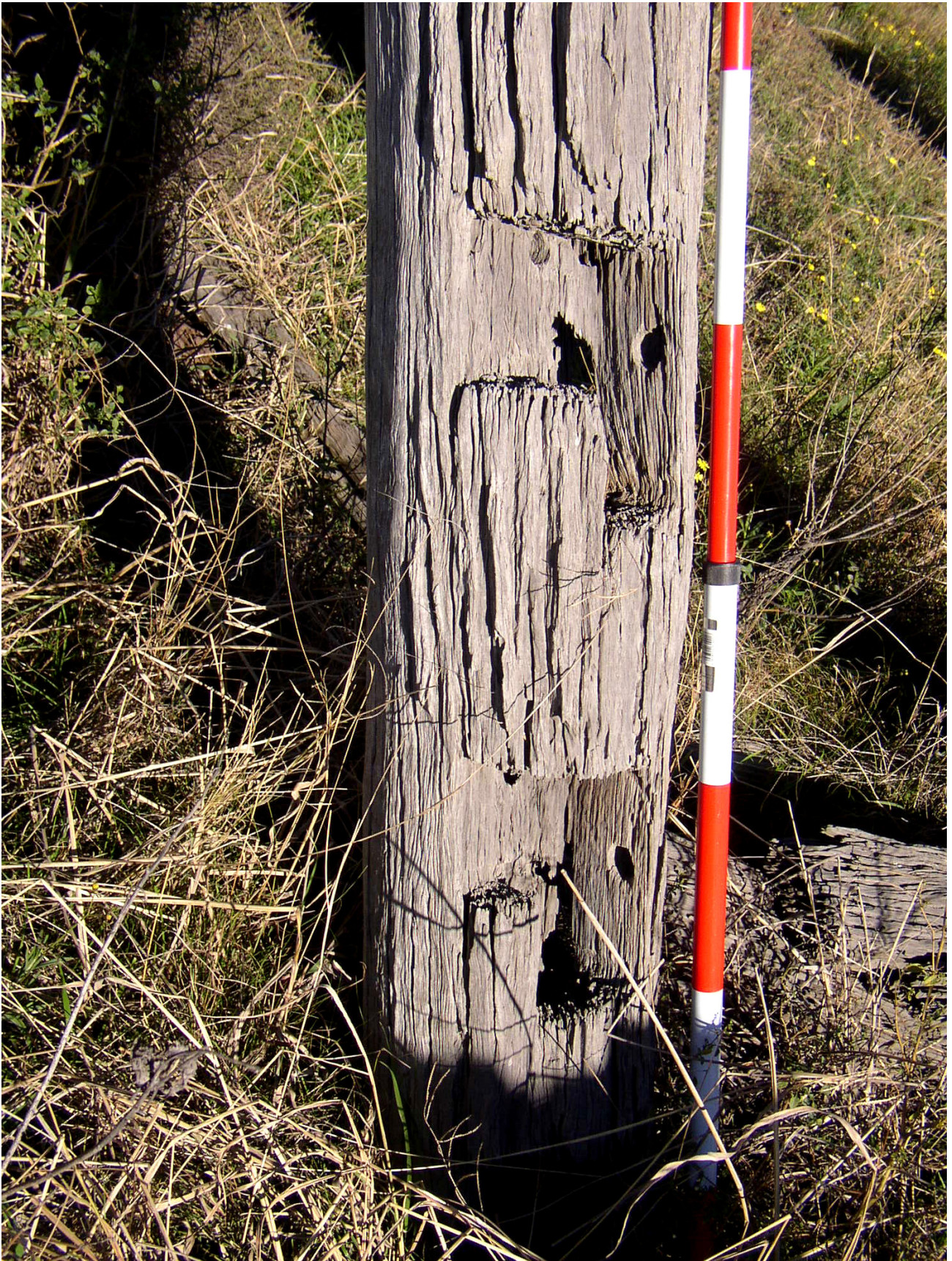
Photo 13. Shows arrangement for slip
