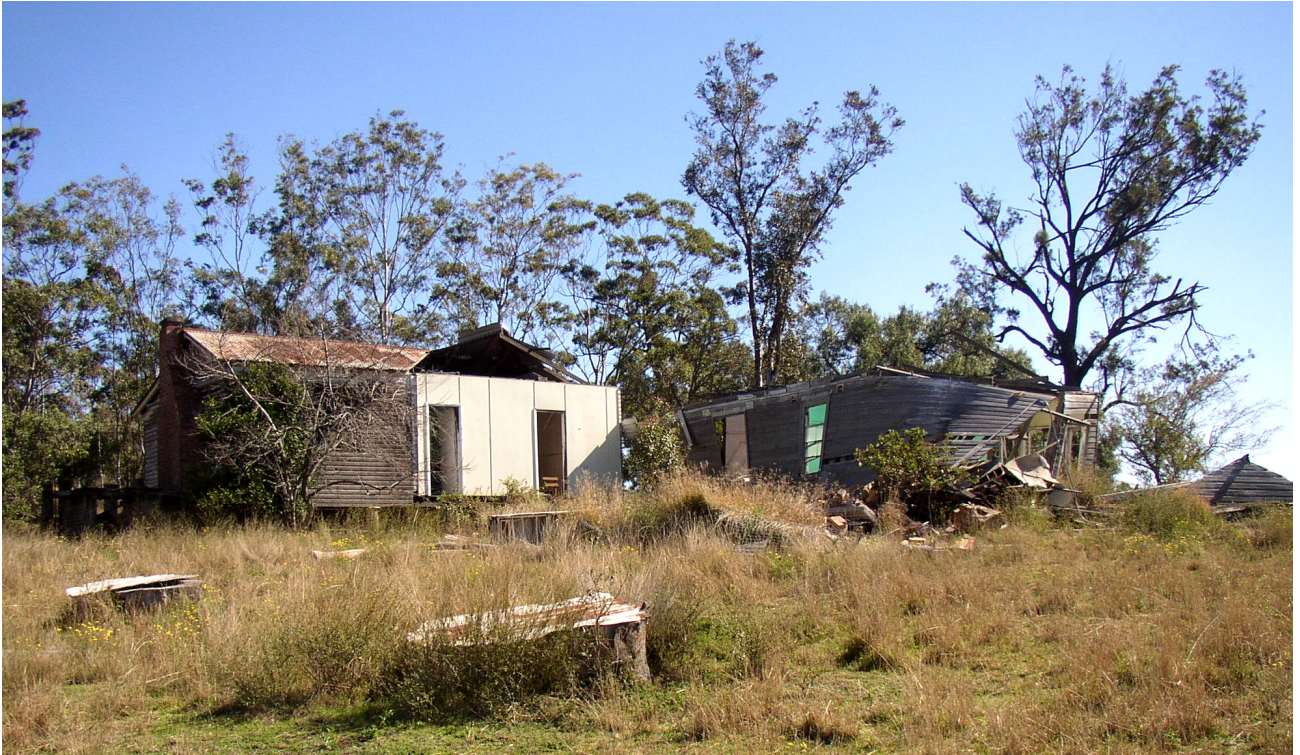
Photo 20 Shows front section of house off piers.
