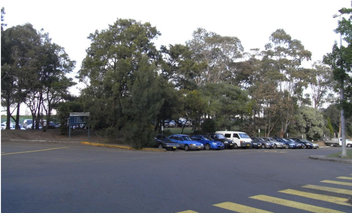
Figure 3: Illustrating the access roads, carparking and landscape plantings in part of the site.
