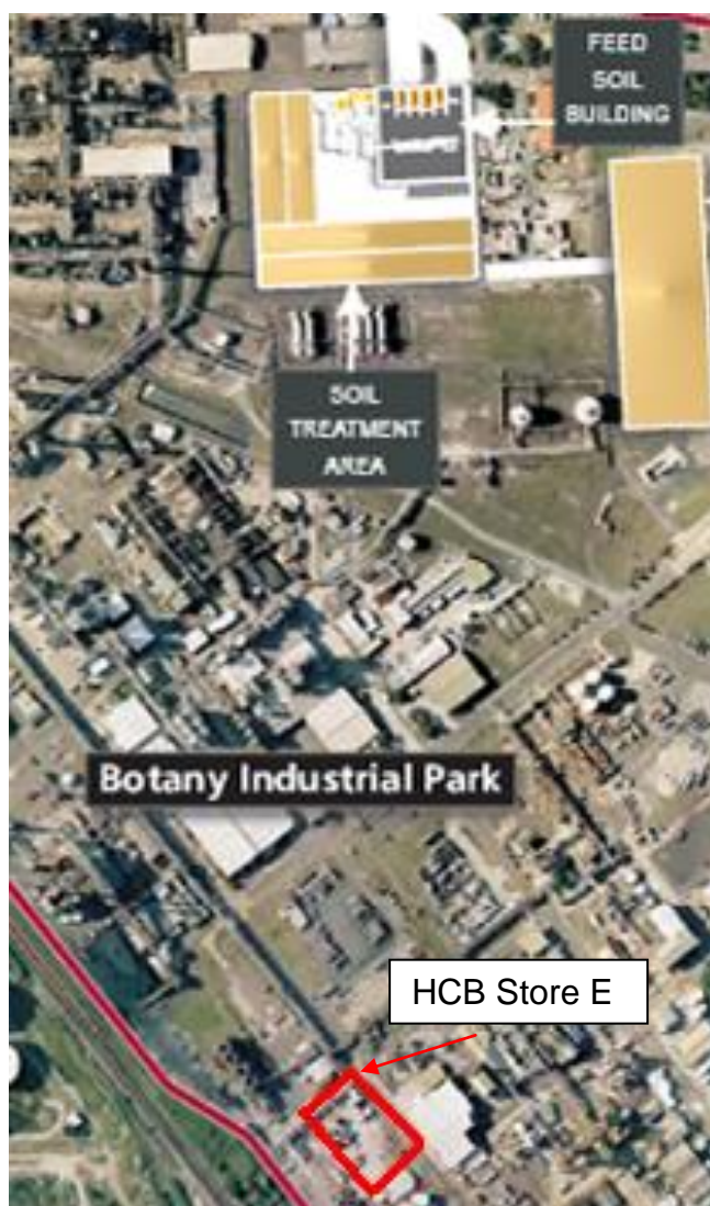
Figure 4-1: Aerial view of the CPWE Remediation Project and HCB Store E.
