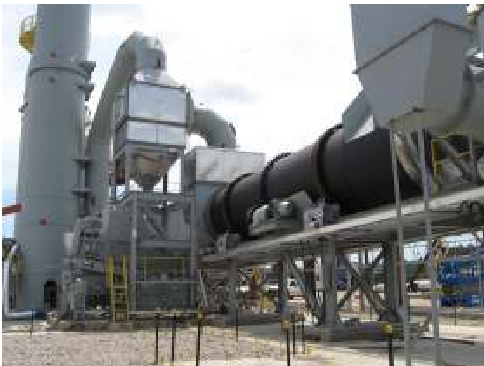
Figure 5 – DTD plant under construction at Rhodes
