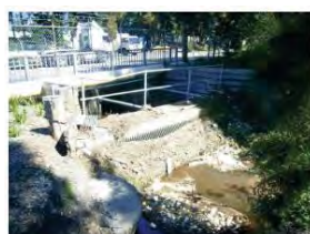
Photo 2: Floodable drain at McPherson Street culvert looking south.
