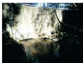
Photo 5: Floodable drain at SWOOS crossing looking south.
