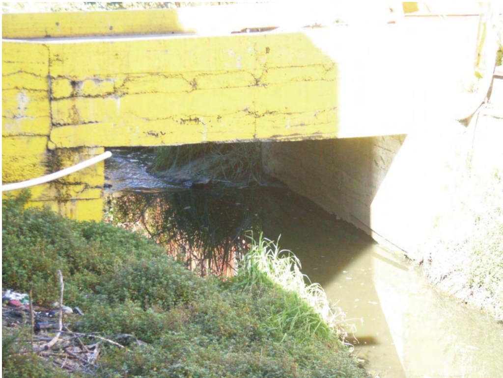
Photo 12: Springvale drain at Bridge 2 looking south.
