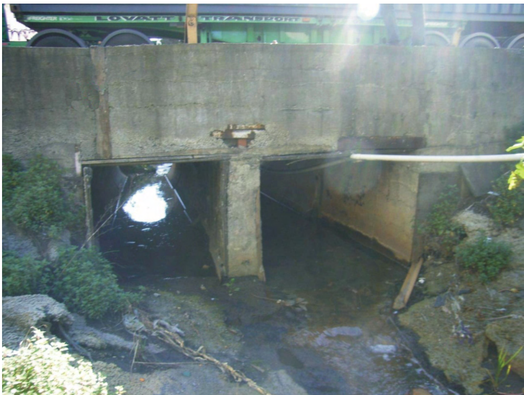
Photo 11: Springvale drain at Bridge 1 looking north.
