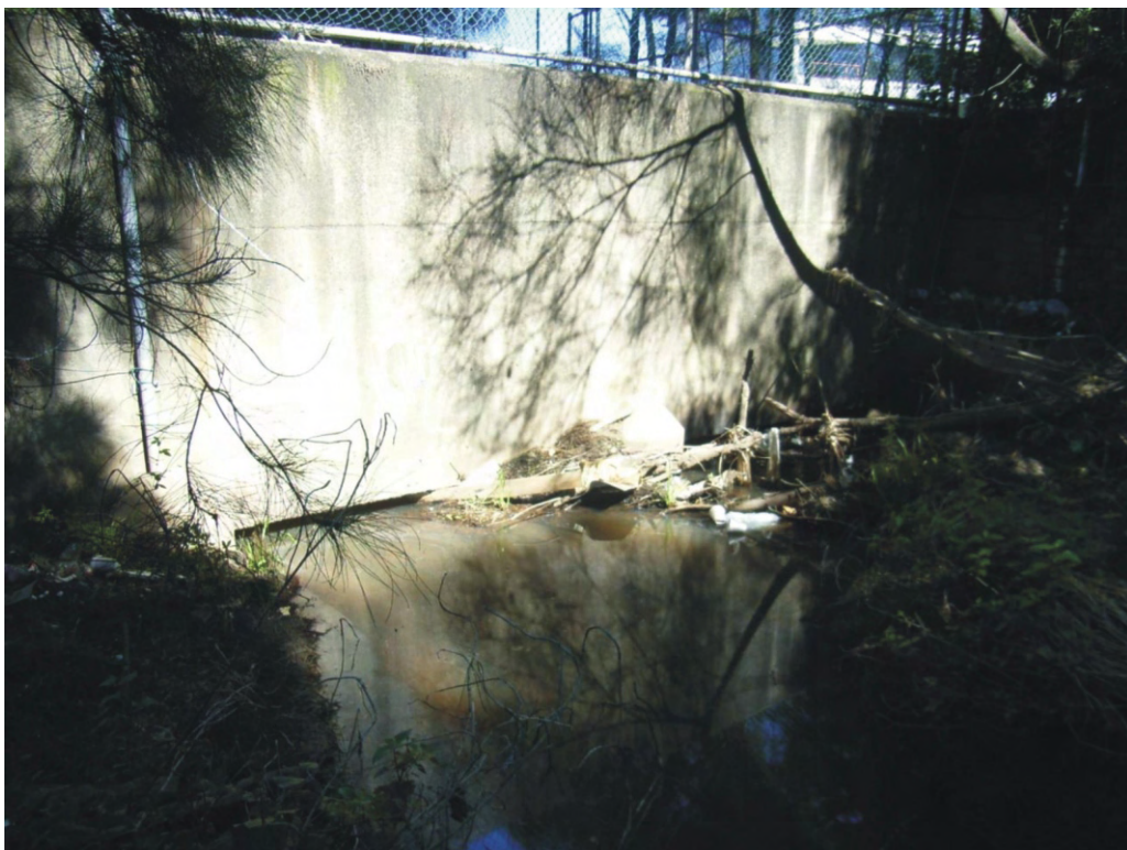
Photo 5: Floodvale drain at SWOOS crossing looking south.
