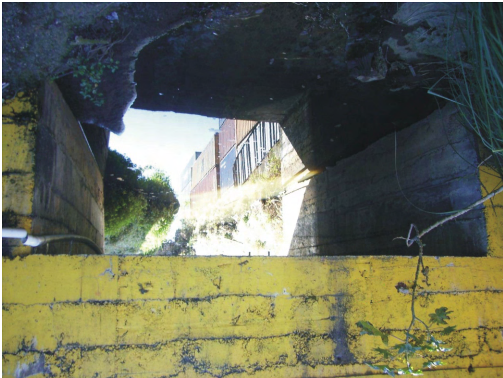
Photo 13: Springvale drain at Bridge 2 looking north.
