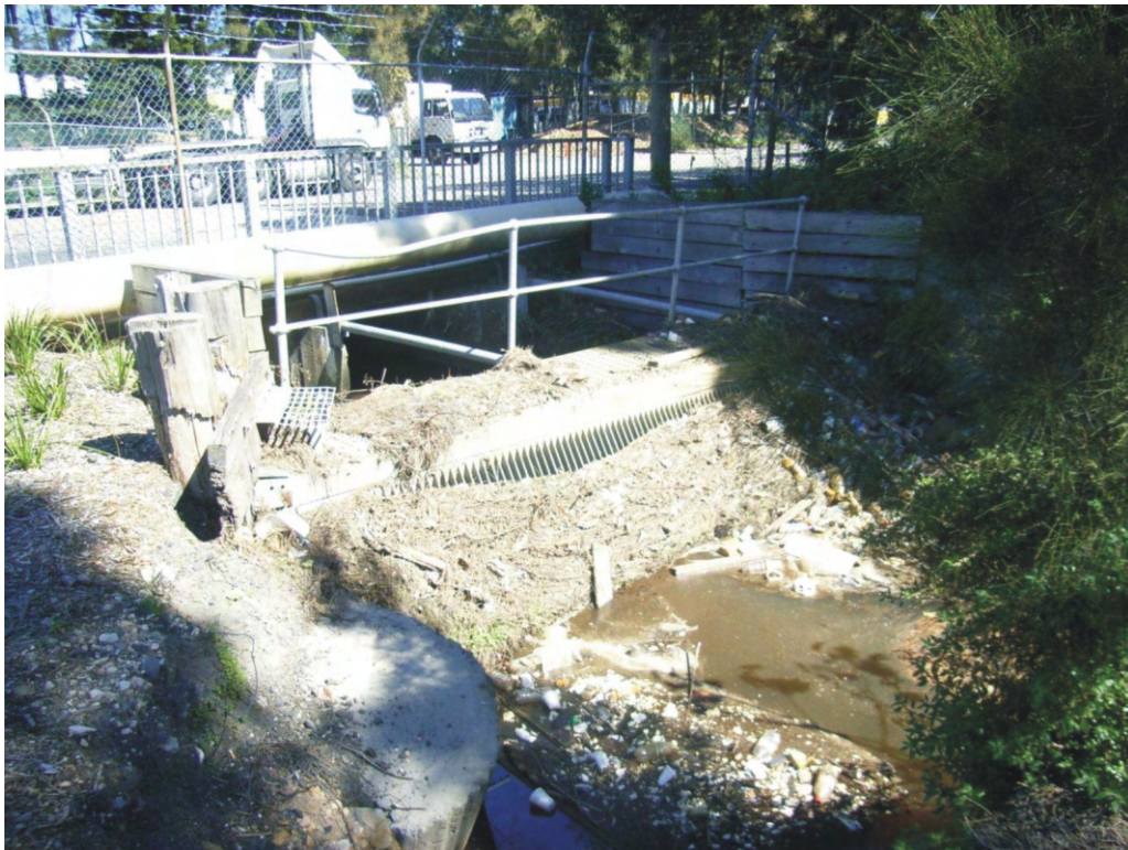
Photo 3: Floodvaley drain at McPherson Street culvert looking south.
