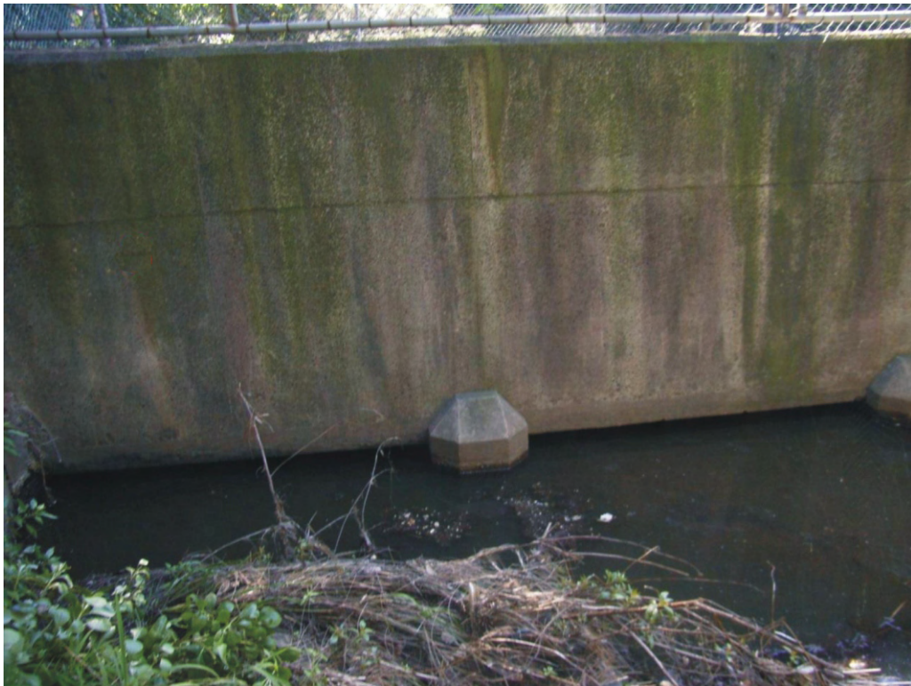
Photo 6: Floodvale drain at SWOOS crossing looking north.
