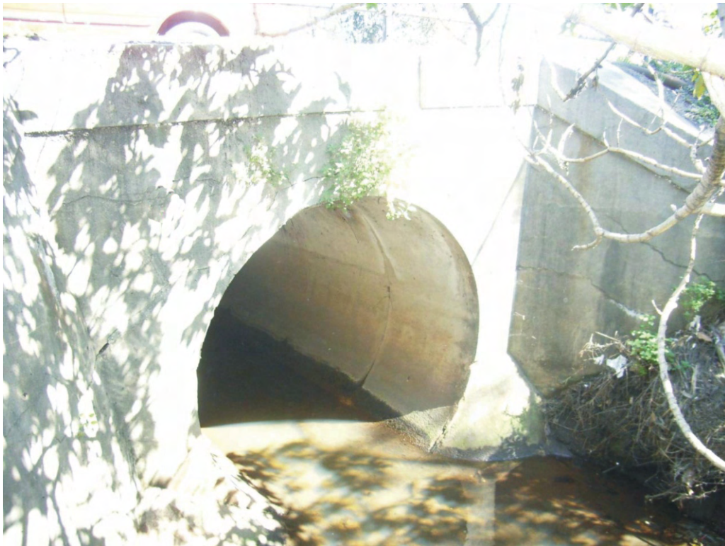
Photo 7: Floodvale drain at Botany Road looking south.
