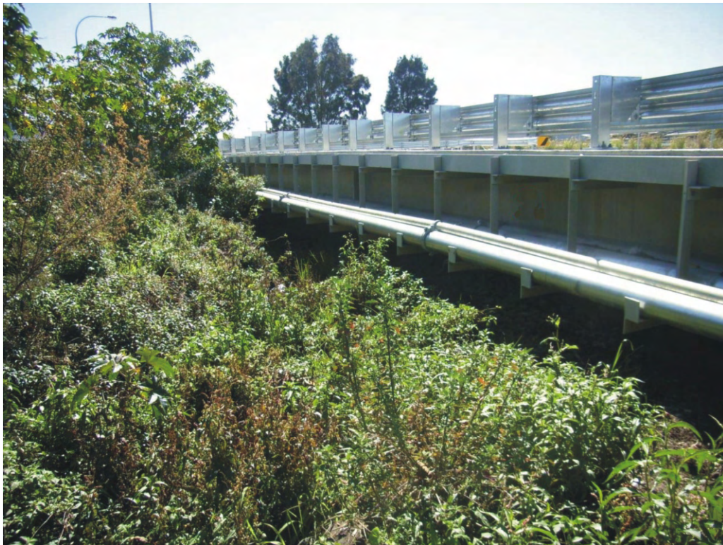
Photo 2: Floodvale drain looking north over Port Feeder Road.
