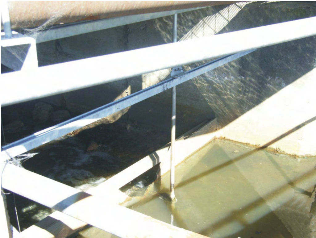
Photo 3b: Springvale drain at McPherson street culvert V notch weir looking south.
