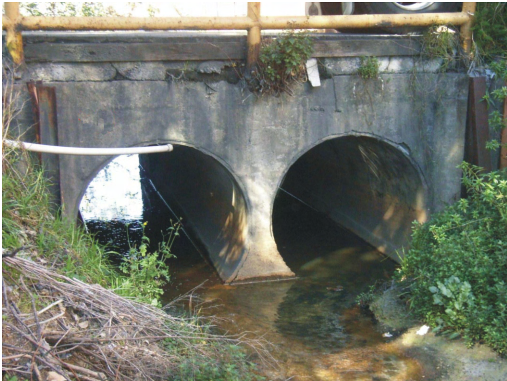
Photo 10: Springvale drain at Bridge 1 looking south.
