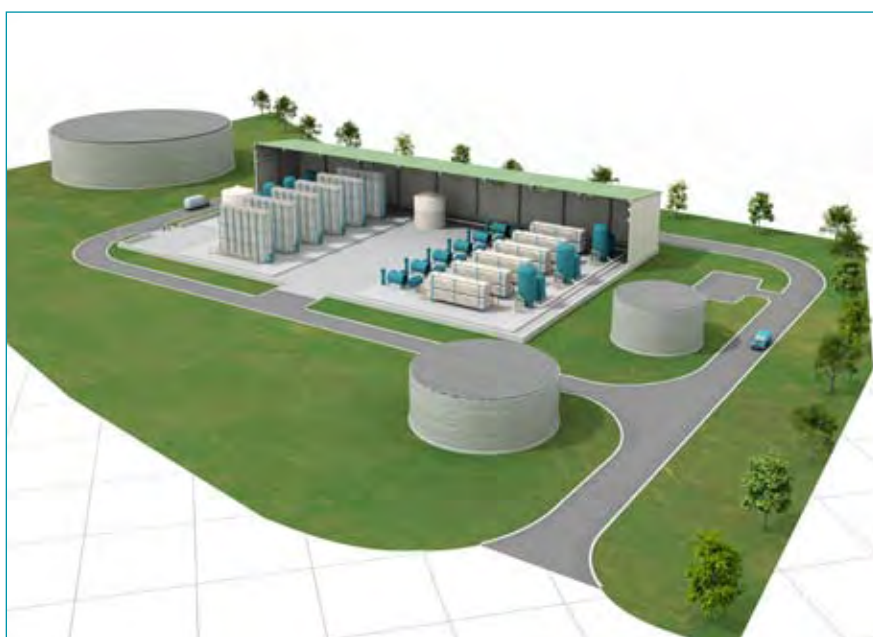
Figure 1.2b Artists impression of AWTP showing internal layout
