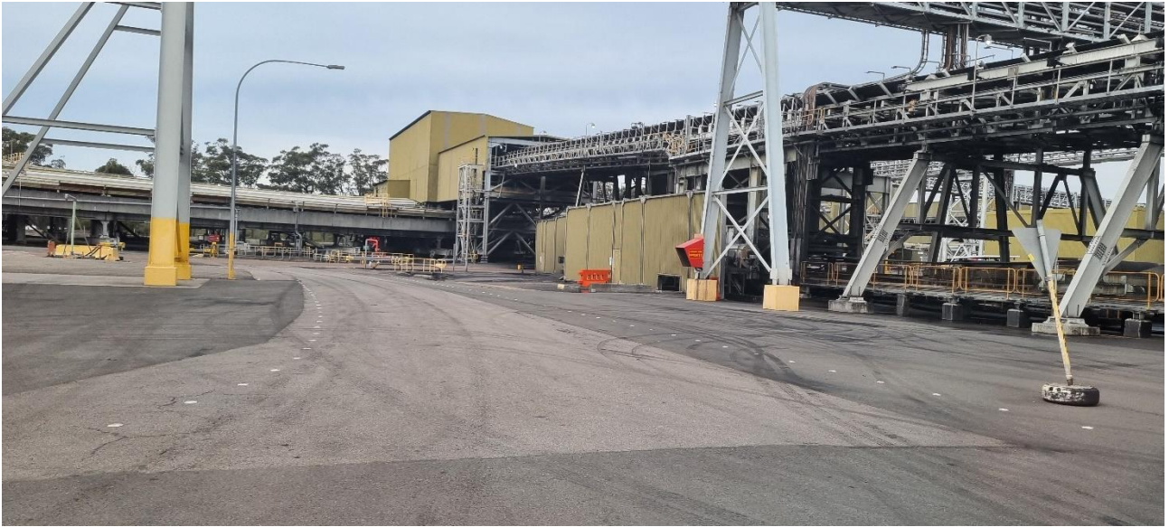
Photograph 4 - Typical Sealed area under coal conveyers
