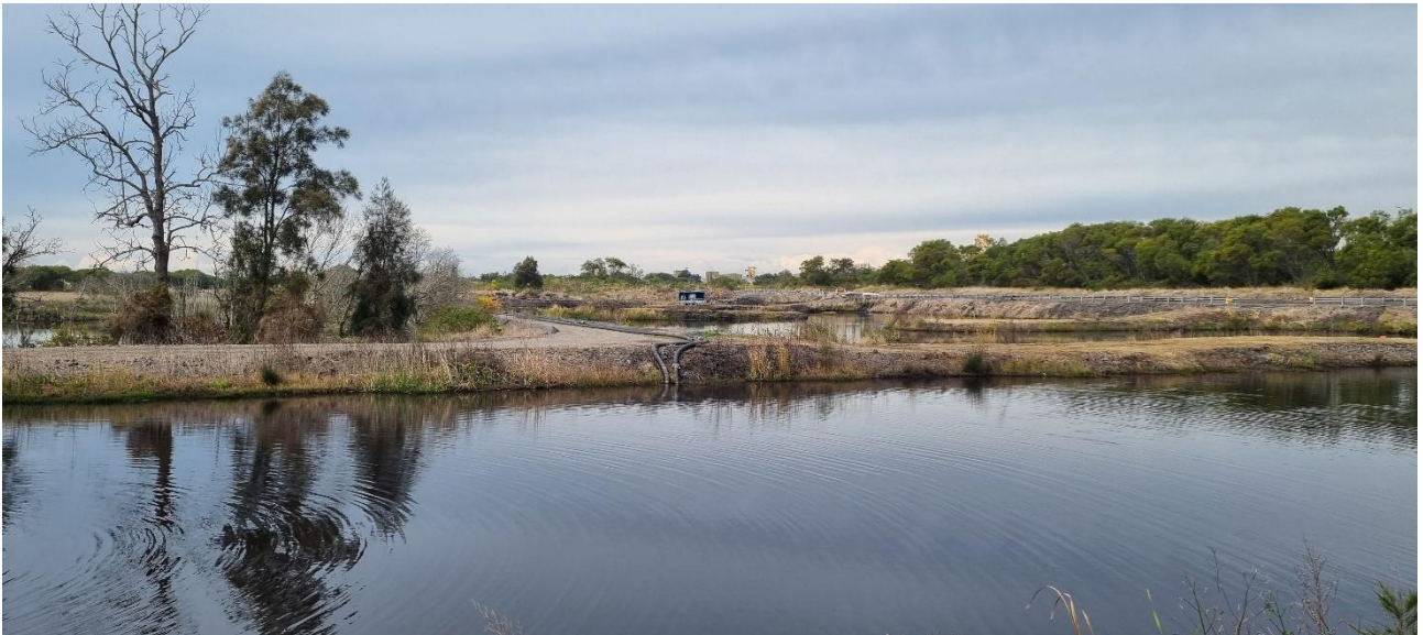
Photograph 3 - Surface Water Detention Basins
