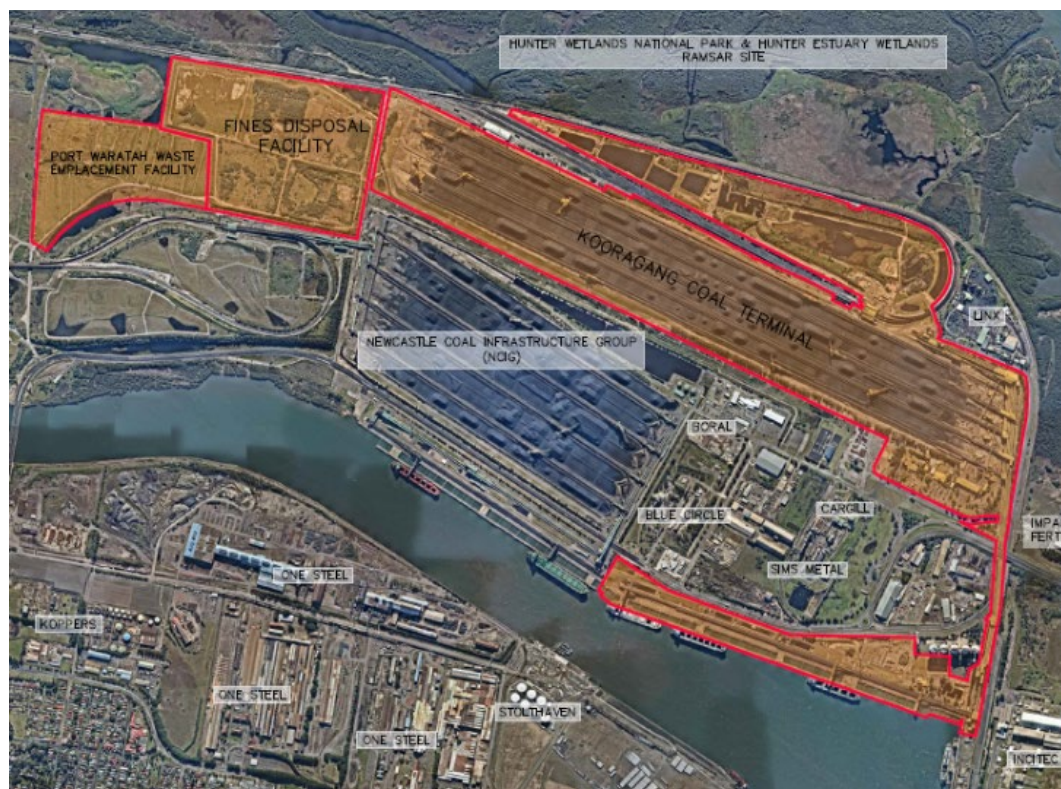
Figure 1: Aerial overview of Kooragang Coal Terminal
