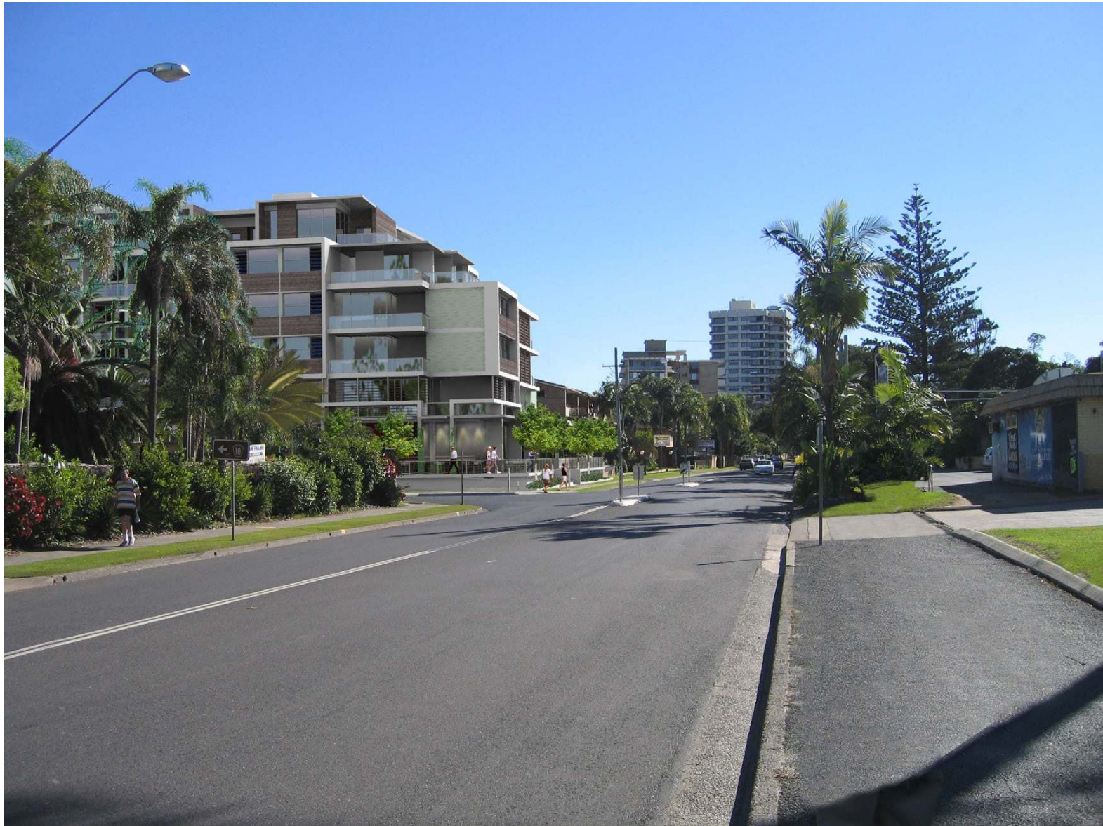
VIEW LOOKING NORTH AFTER
