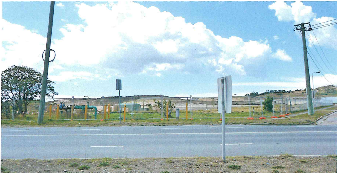
Figure 3: View of Cell 1 from the entry road to the site, at RL 37.15 (photo taken 8 October 2013)
