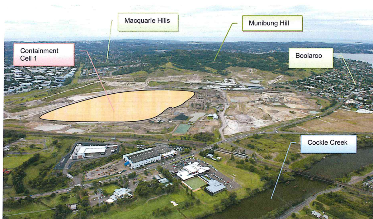
Figure 2: Aerial view of the Pasminco site and surrounds, with the containment cell (Cell 1) in the centre
