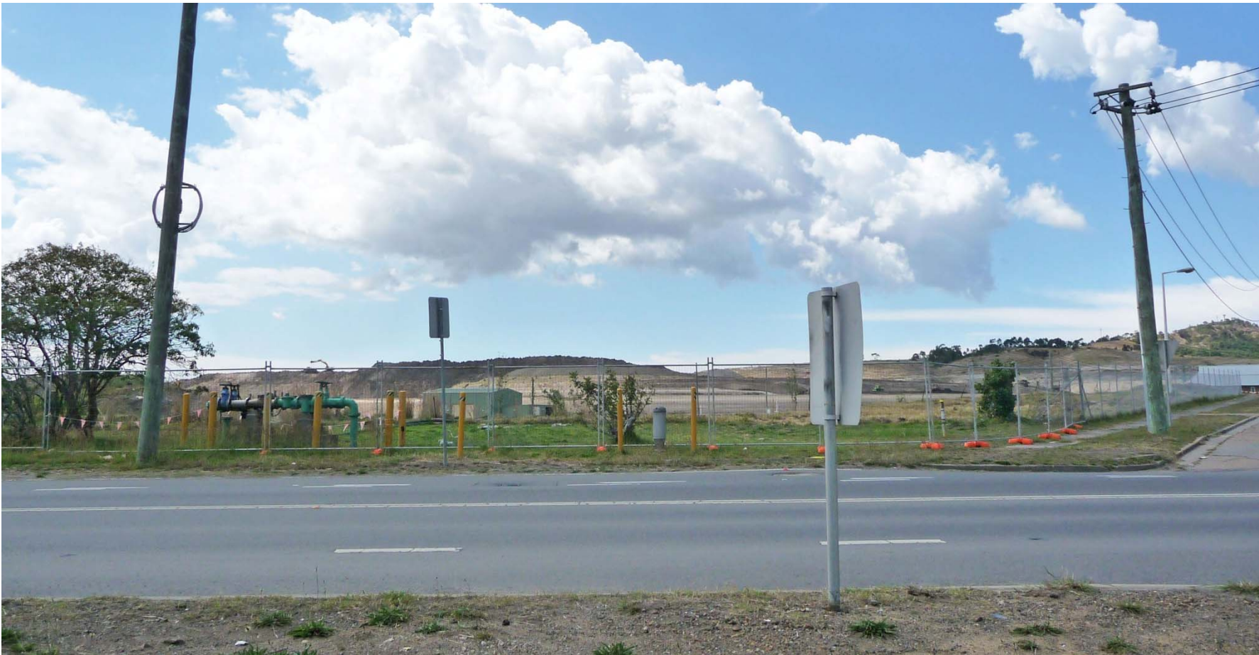
Photo 1A View of the site and containment cell from entry road to Cockle Creek railway station, with cell platform at approx. RL 37.15 (as advised), with temporary stockpiles located on the cell platform (8 October 2013)
