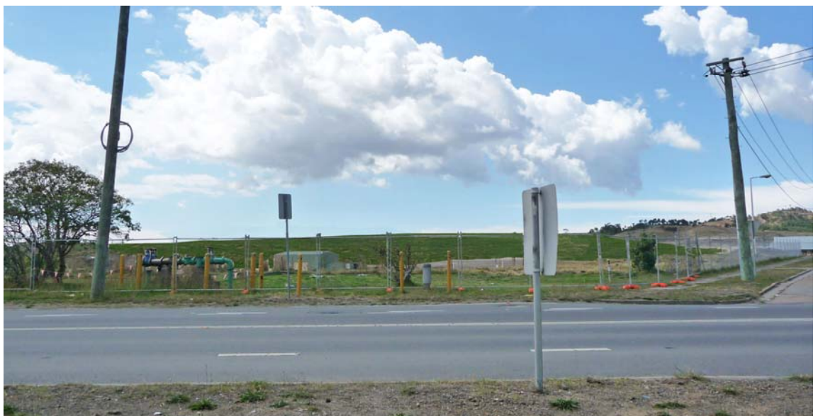
Photo 1B: Photomontage of the same view of containment cell with height of cell raised by up to 4.15m (from its approved RL 38.0 to RL 42.15), with landscape cover over cell and slopes
