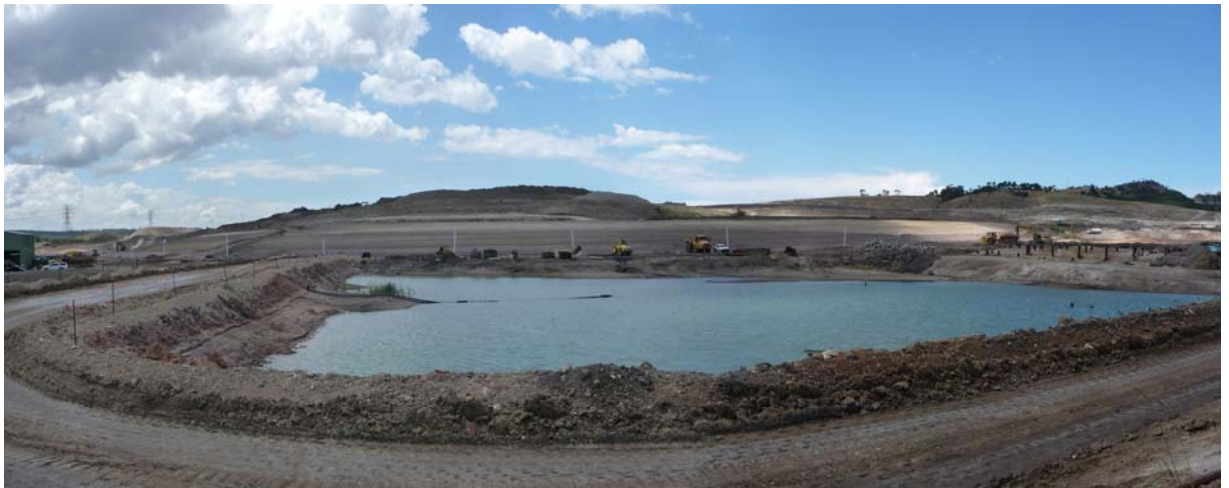
Photo 6A: View of the containment cell constructed to RL 37.15 (as advised) from location adjacent to the former Laboratory building, with temporary stockpiles on the cell platform (October 2013)
