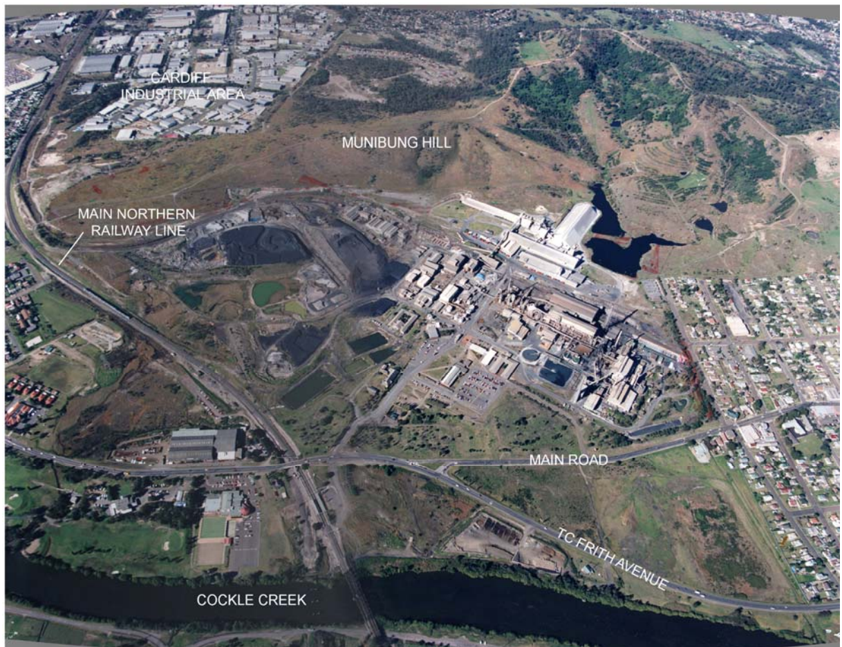
Figure.1: Aerial view from the east of the PCCS and IFL sites, Boolaroo (1998), with industrial buildings on both sites
