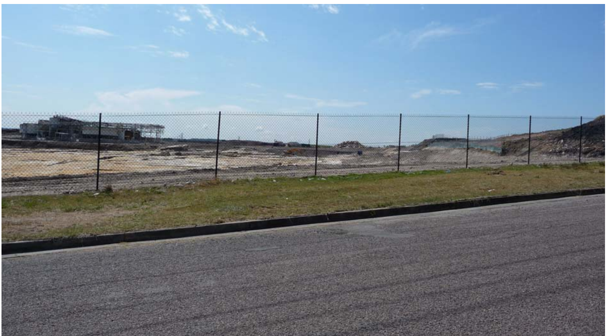
Photo 5B: View north-east to the PCCS site from First Street, Boolaroo
