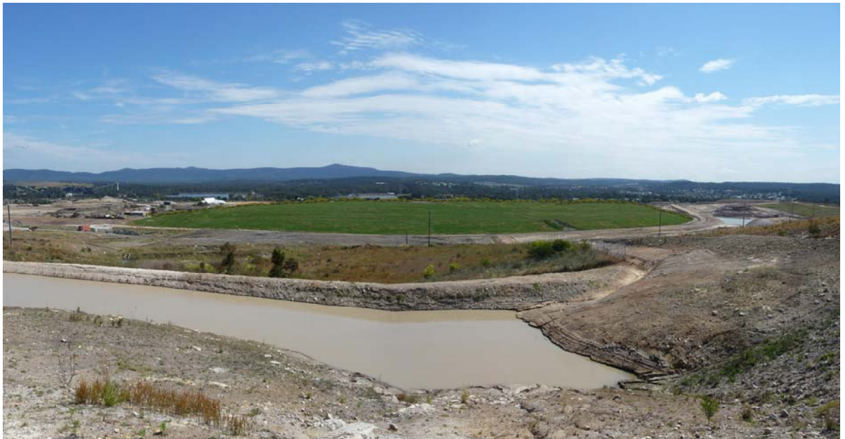
Photo 4B: Same view of the containment cell with height of cell raised by up to 4m (up to RL 38), with landscape cover over cell and slopes
