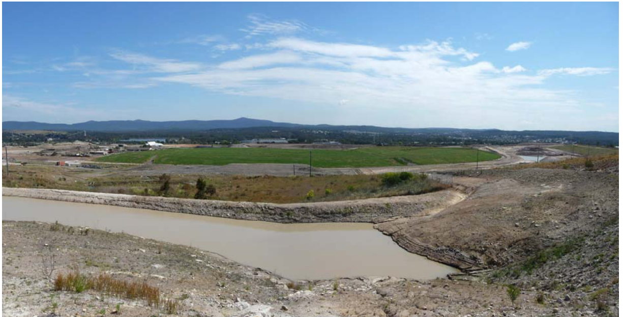
Photo 4A: View of site and containment cell from Munibung Hill, east of the site
