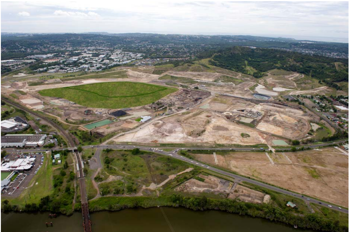
Photo 9C: Aerial photomontage of a single containment cell from the west, with height of cell raised by approx. 4m (to RL 38), with landscape cover over cell and slopes. Usable open space delineated by proposed ring of vegetation.
