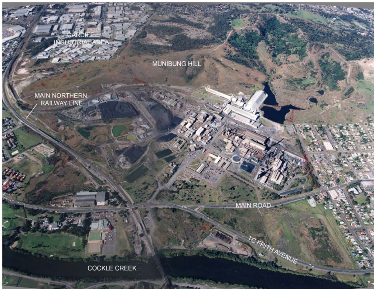
Figure 1: Aerial view from the east of the PCCS and IFL sites, Boolaroo (1998), with industrial buildings on both sites
