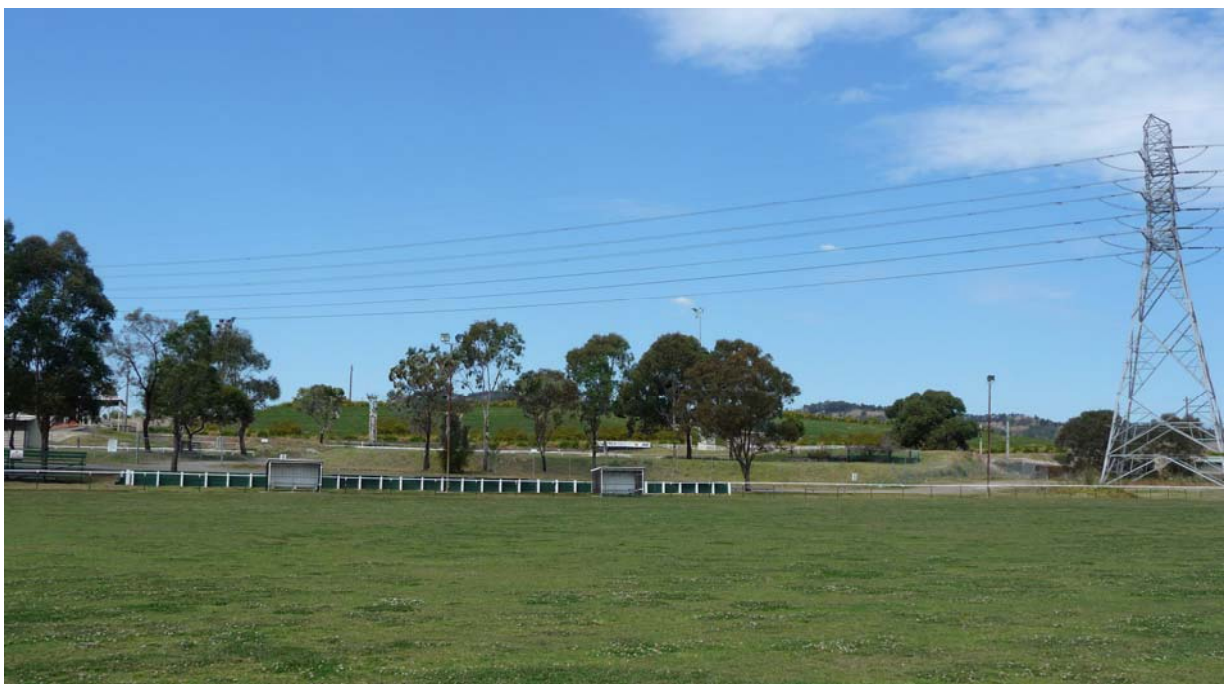
Photo 2B: Same view of the containment cell with height of cell raised by up to 4m (to RL 38), with landscape cover over cell and slopes
