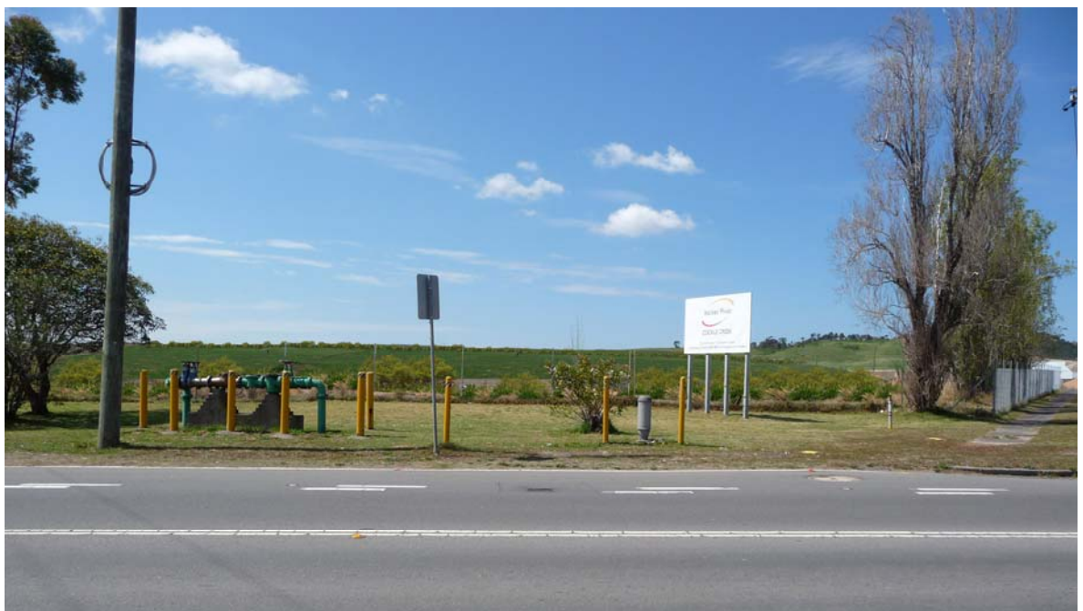
Photo 1B: Same view of containment cell with height of cell raised by up to 4m (to RL 38), with landscape cover over cell and slopes
