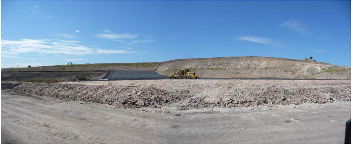
Photo 7A: View of the containment cell from within the site
