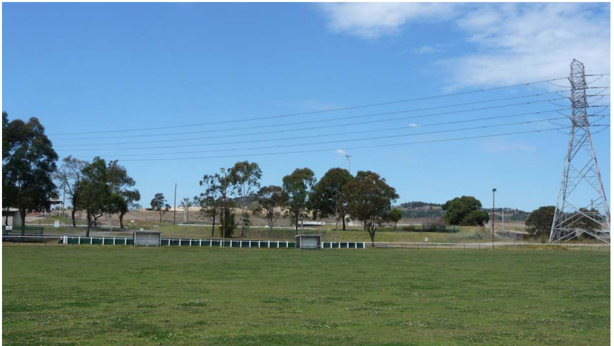
Photo 2A: View of site and containment cell from Jack Edwards Oval, west of the site
