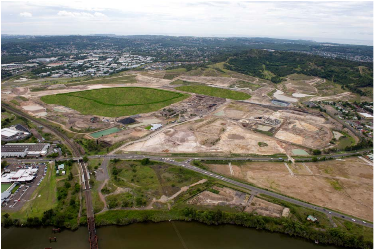
Photo 9B: Aerial photomontage of the proposed PCCS and IFL containment cells from the west, as approved with usable open space at the top of the cell delineated by the proposed ring of vegetation.
