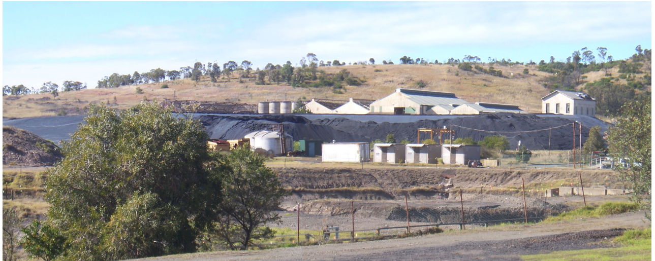
Photo 10A: View within the PCCS site behind the former Laboratory building, northwards towards the cell structure with existing buildings to be demolished.
