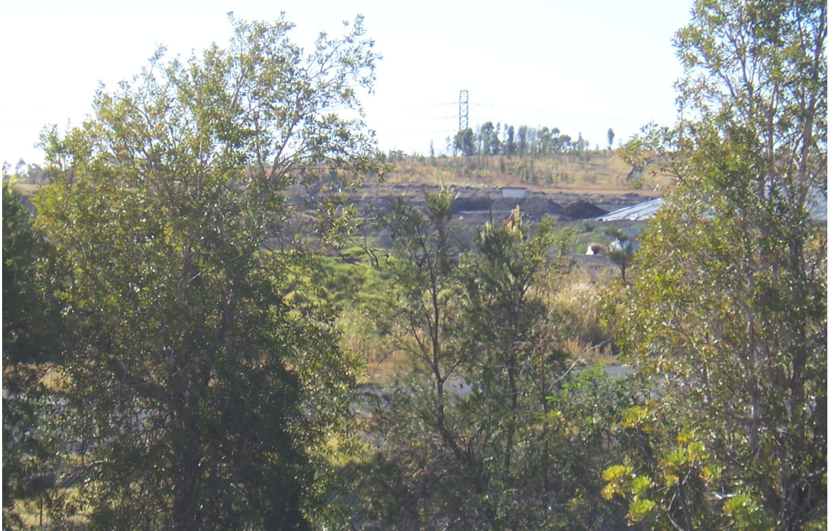
Photo 11A: View from PCCS site, towards the existing cell structure
