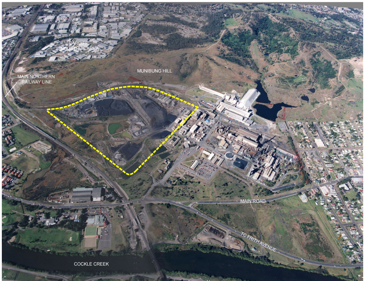
Figure 3: Aerial view of the PCCS site illustrating proposed footprint of future cell (shown dotted)
