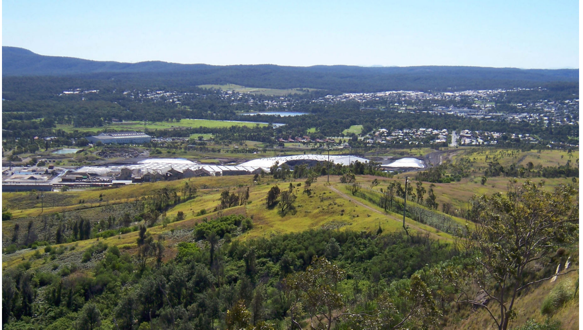
Photo 8A: View of the site and existing cell structures from the upper ridges of Munibung Hill, to the east. Buildings in the cell foreground will be demolished.
