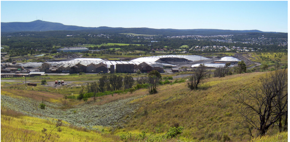
Photo 9A: View of the site and existing cell structures from the lower slopes of Munibung Hill, to the east. Buildings in the foreground of the cell will be demolished.
