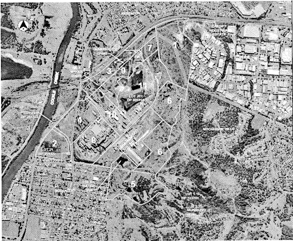
Figure 1 – Aerial Photograph of the PCCS Site divided into numerical Work Areas
