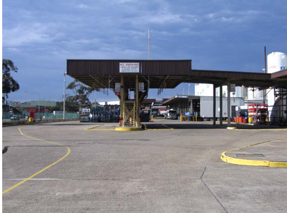
Photo 2 – Existing Vopak Site A – Internal Operation
