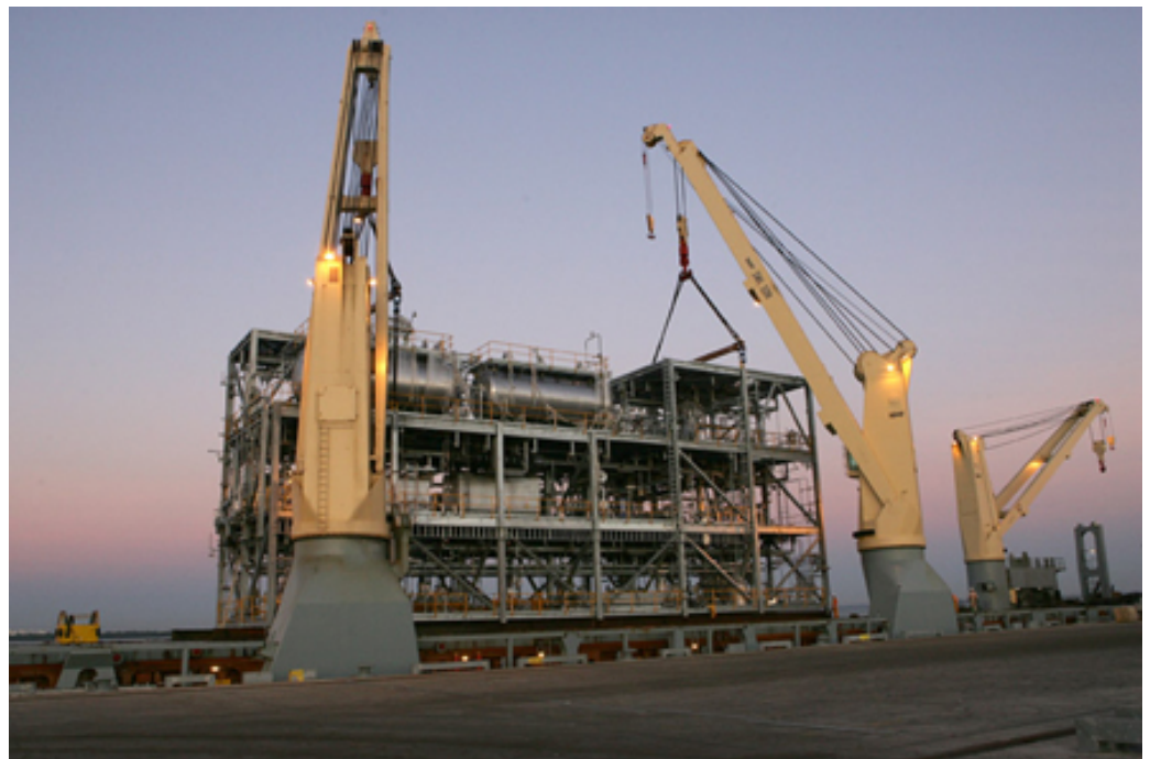
Figure 7.5 The use of construction cranes at the Darwin biodiesel plant
