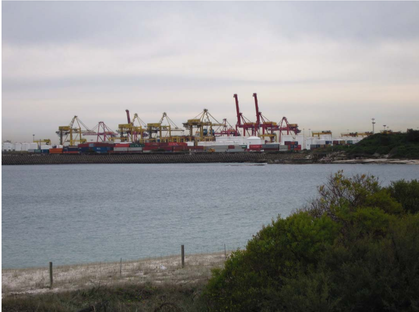
Figure 7.6 Vopak Site A, when looking from Yarra Bay sailing club (photo: Vopak 2006)
