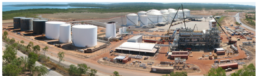
Figure 1.1 Darwin biodiesel plant under construction (July 2006) (Source NFAL)
