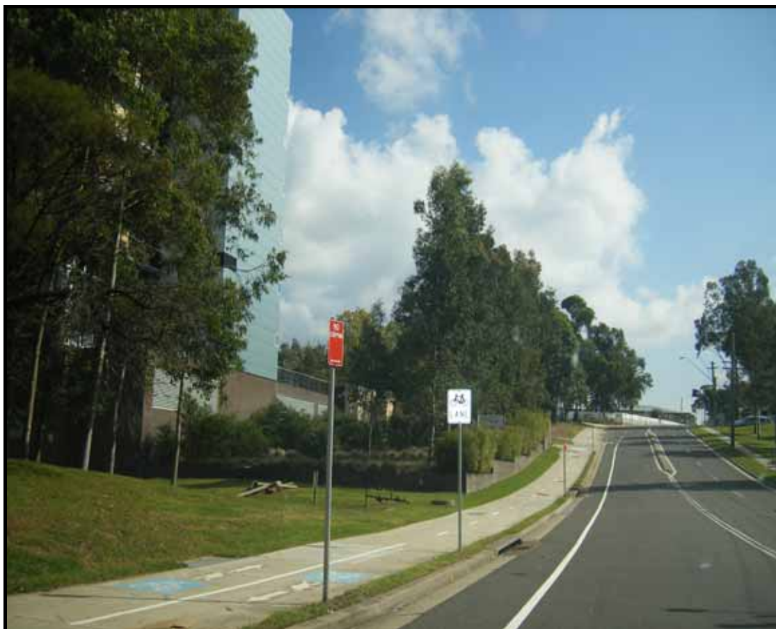
Figure 12 – View of existing Talavera Road setbacks and condition
