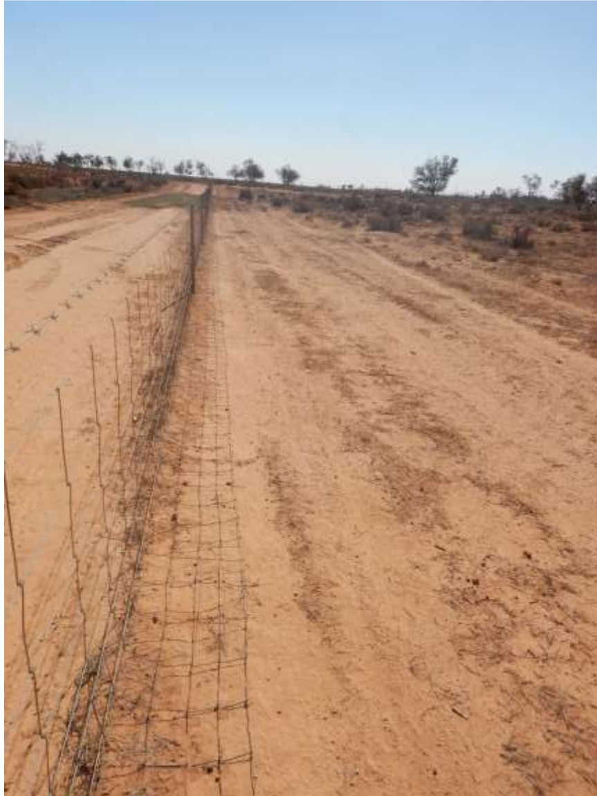
Apron attached to bottom of fence
