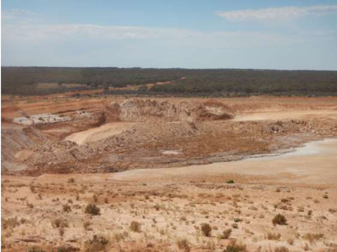
Capping of slimes with overburden at the former water dam (2018)
