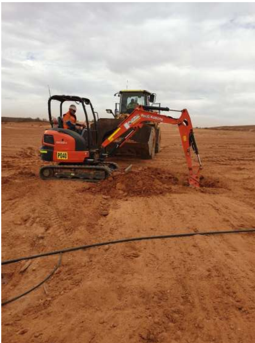
Tree wells being excavated with a 3 tonne digger
