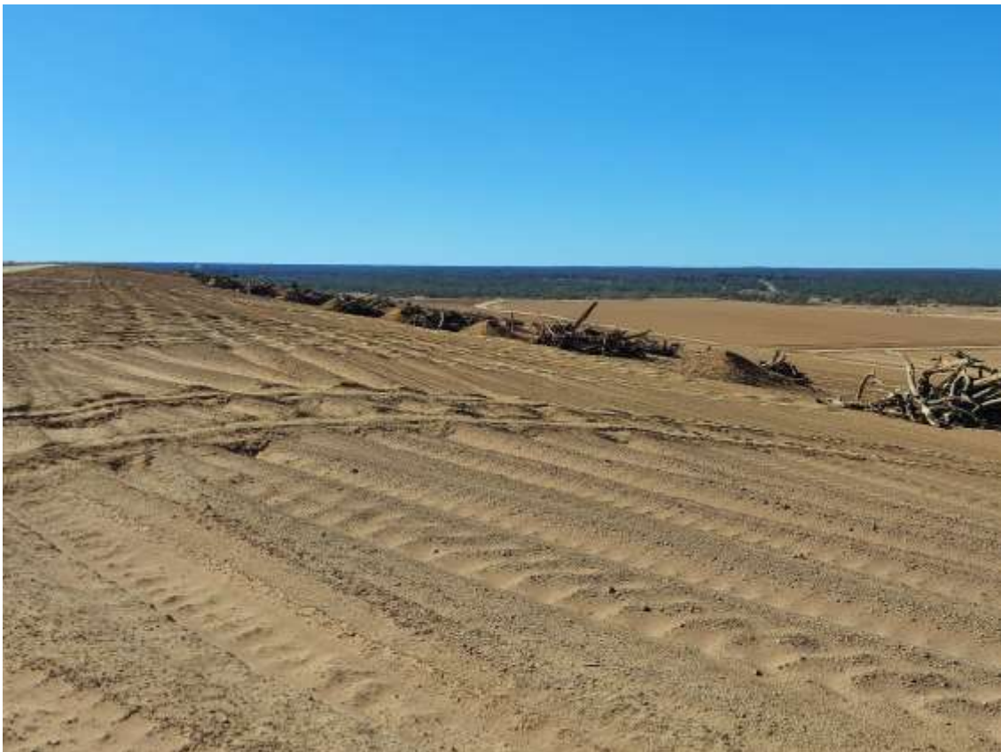
Final landform topsoiled and timber being placed onto batters. (July 2020)
