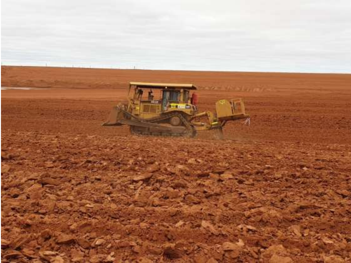
D9 dozer with Gessner drum seeder mounted above 3 rippers.
