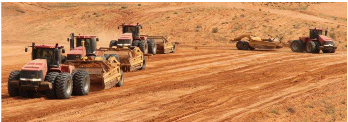
Tractor and scoops used for topsoil and subsoil stripping and replacement
