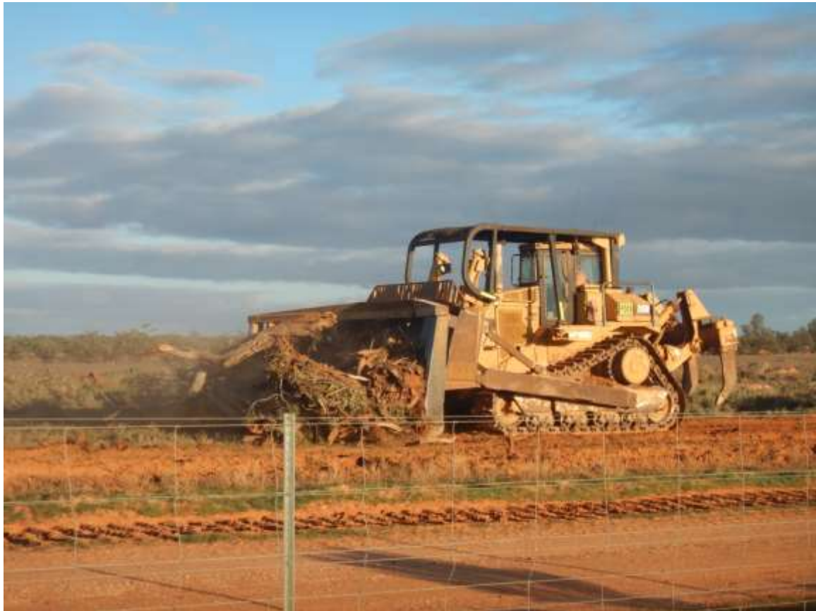
Vegetation being pushed into windrows to be used in future rehabilitation
