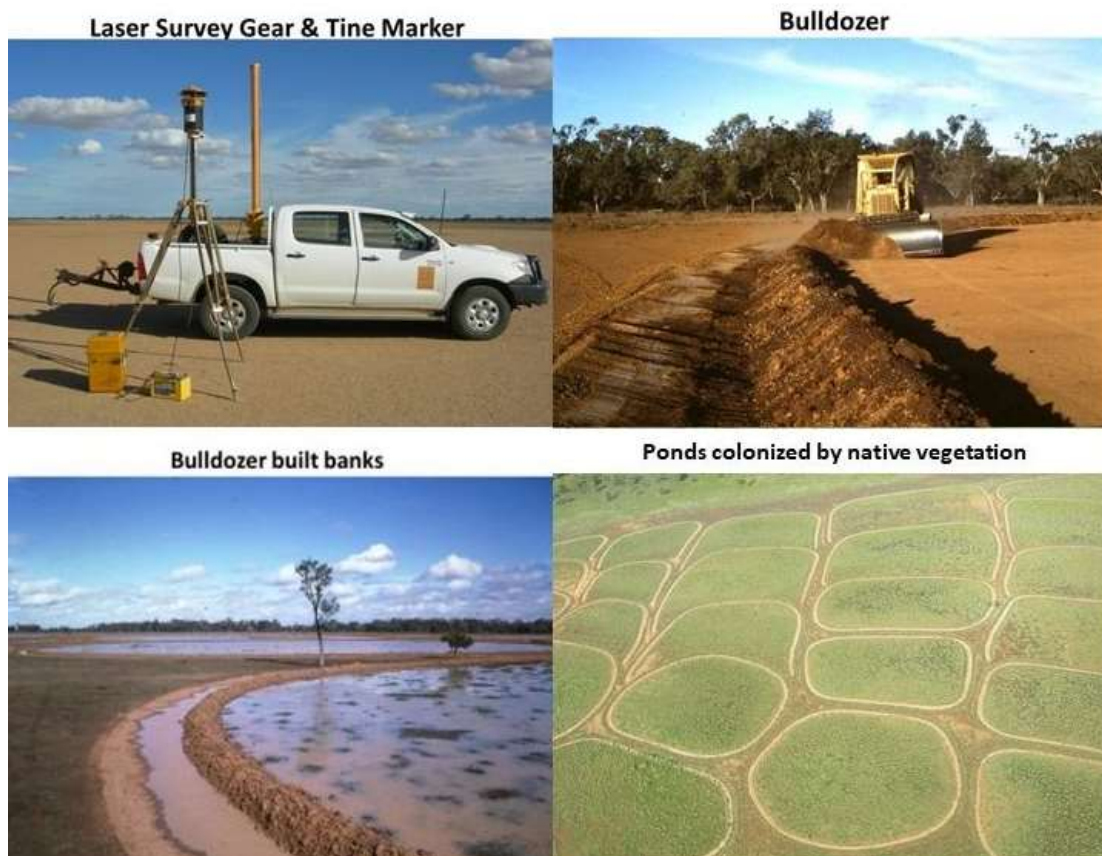
Construction of mini catchments by NSW Local Land Services
