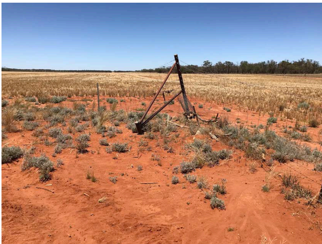
Photo 10 Damaged fence corner strainer post at south-eastern border of Offset 2 area.
