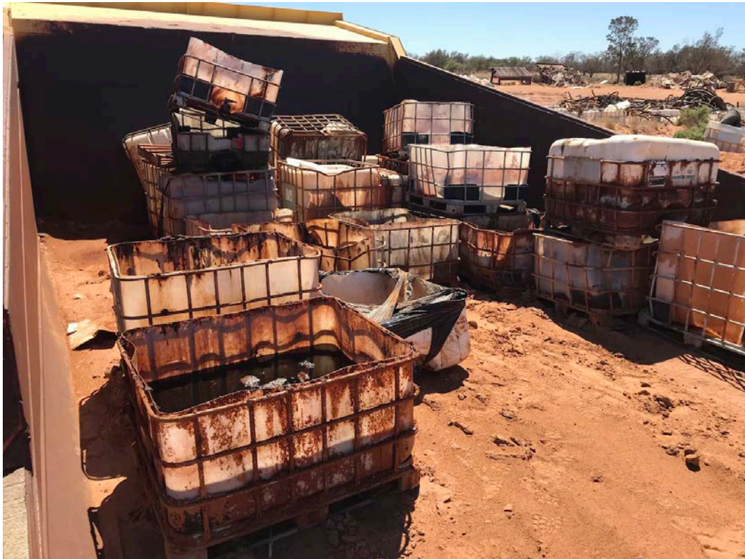
Photo 5 Waste oil stored in open-topped IBCs at BSL compound.
