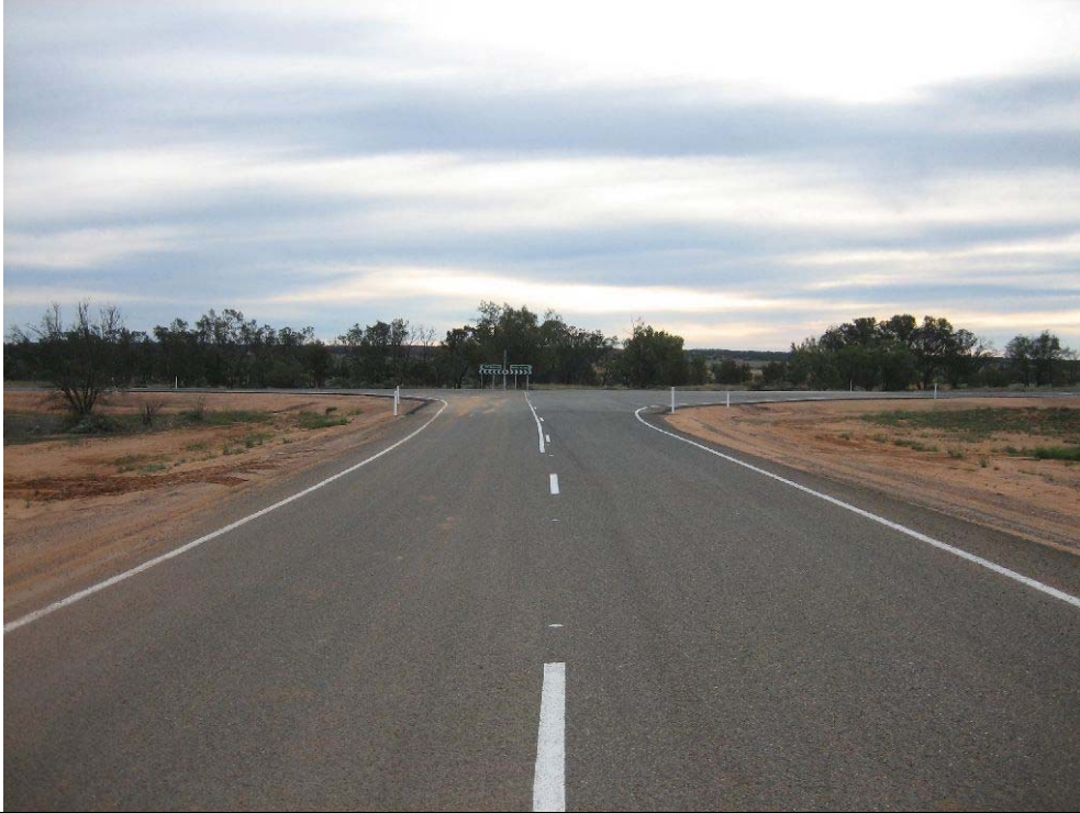
Photo CA-1: View looking west along the existing Ginkgo Mine Highway Access Road (HAR) towards the Silver City Highway. Upgrades by BEMAX have included sealing a short section of the road on approach to the Silver City Highway, as well as right-turn and left-turn improvements to the intersection.
