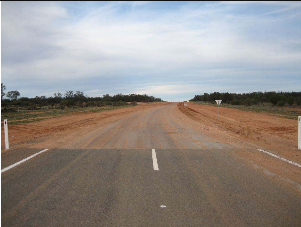
Photo CA-2: View looking east along the existing Ginkgo Mine HAR showing the transition between the sealed and gravel pavements. Upgrades by BEMAX include upgrading an existing section of Old Roo Roo Road, new sections of the road on an improved alignment as well as sealing of a short section of the road on approach to the Silver City Highway.
