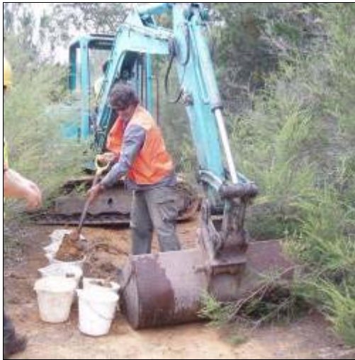
Figure 2.1 Excavating at test pit 18
