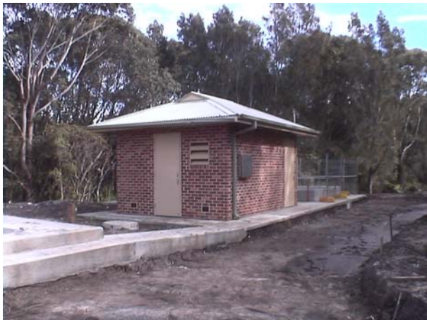
Photo 16: Shoalhaven City Council Sewer Pumping Station
