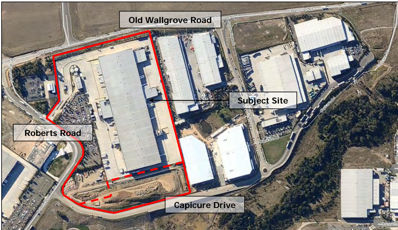
Figure 4. Aerial Photo (showing recent development) (Source: Nearmap, 2012)
