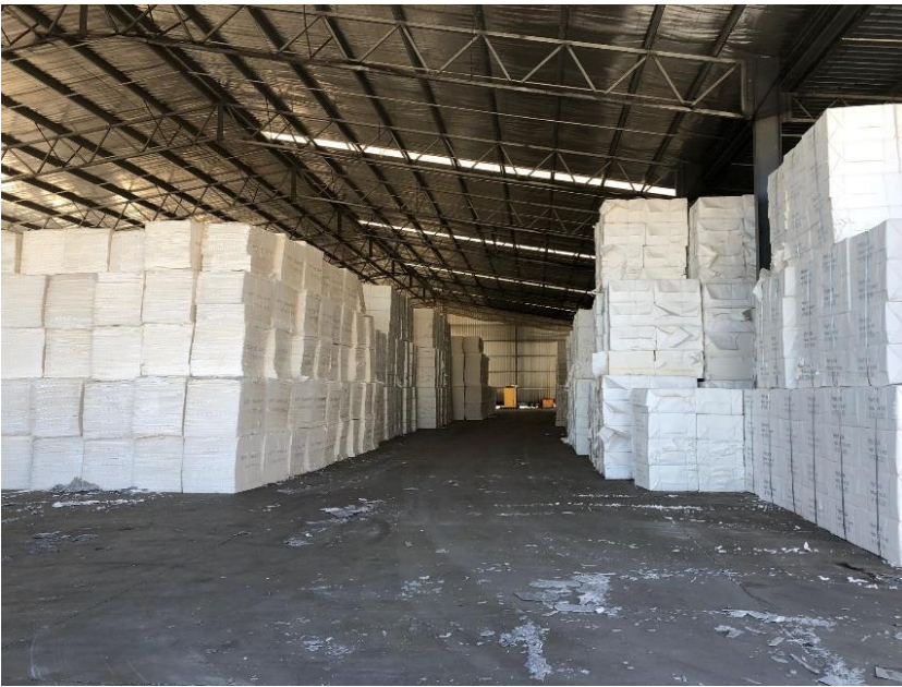
Figure 3.3 Existing BKP shed
