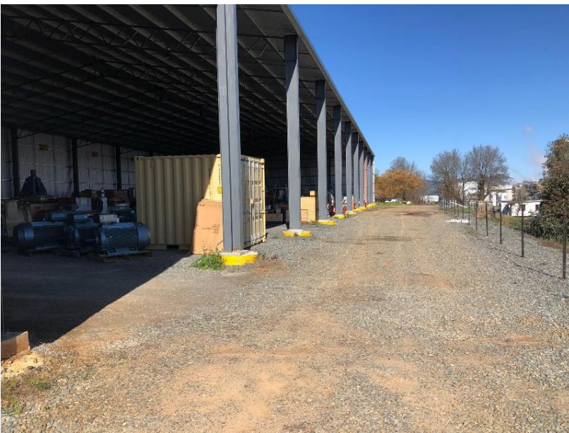
Figure 3.4 Existing storage shed
