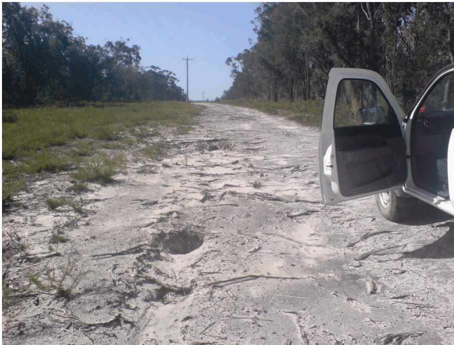
Figure 6 View north along existing transmission line. Notice sandy soils that are exposed to erosive forces.
