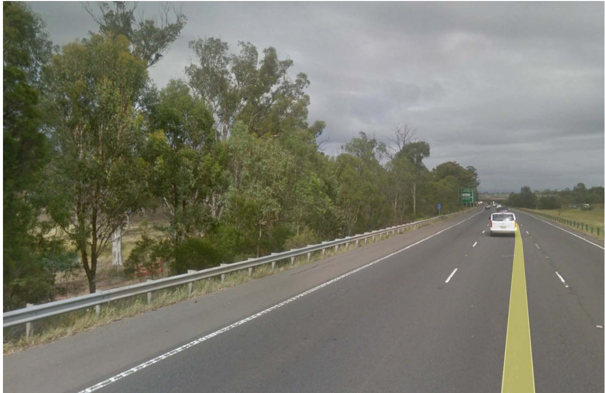
Photograph 7.5 Viewpoint 6 – Western Motorway – Looking south-west
