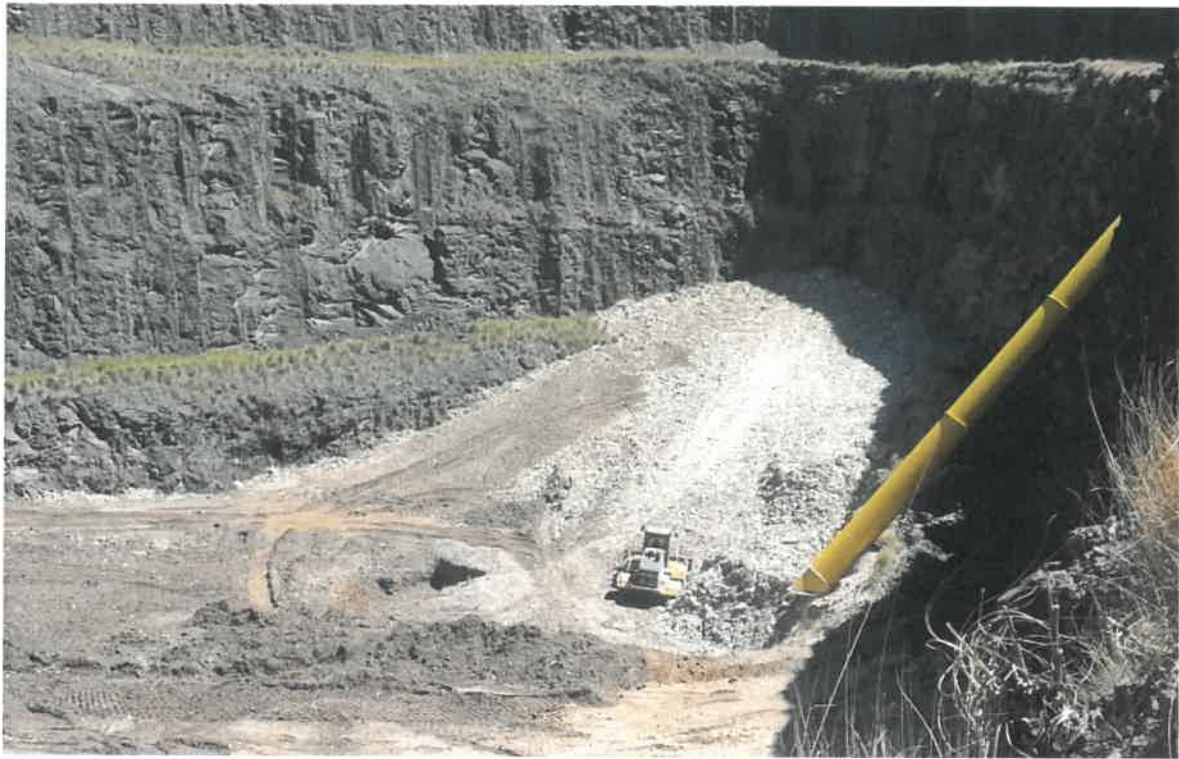
FIGURE 6 – Landfill Operations – chute waste from Genesis MPC
