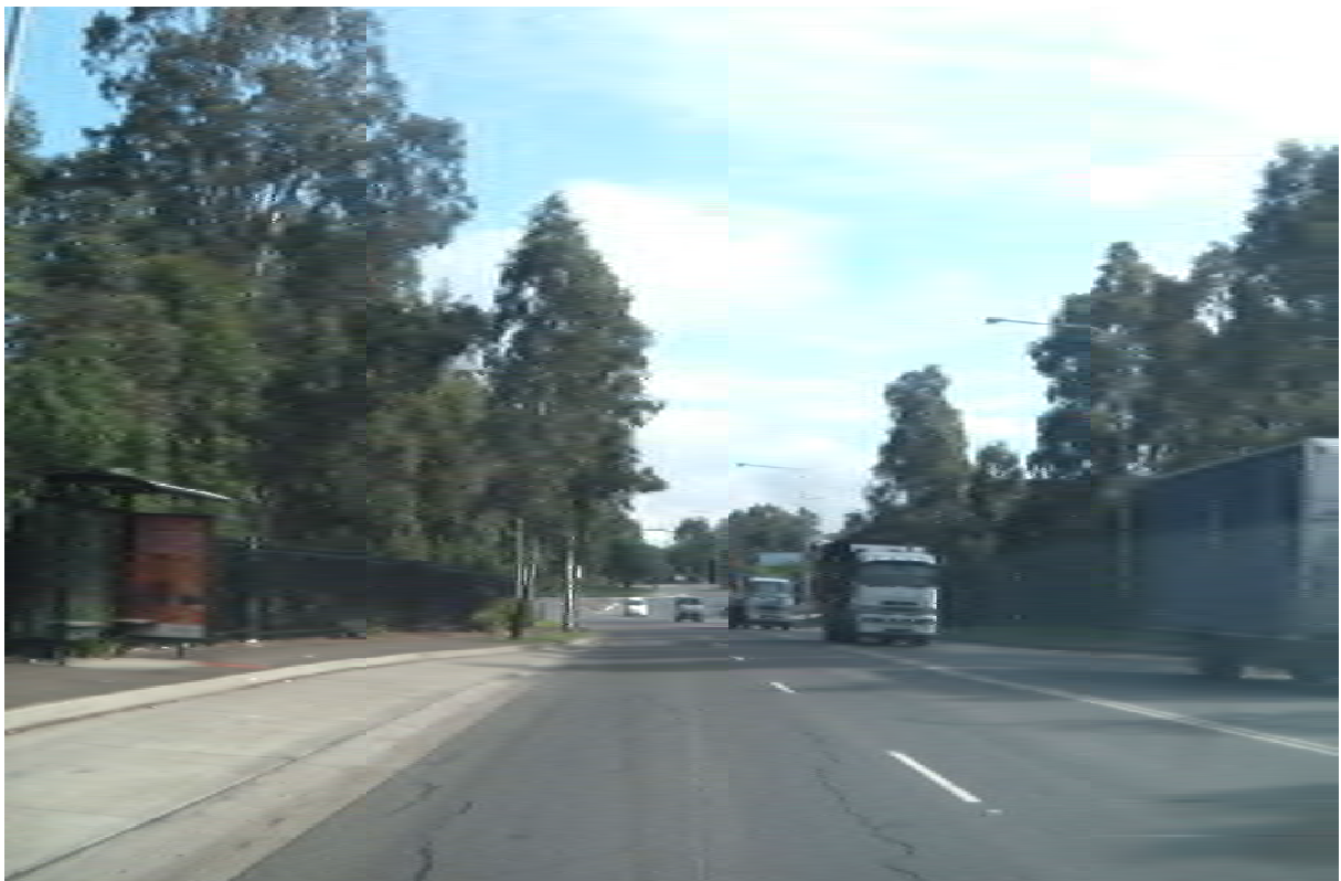
Photograph 2.18 Indented bus bays with bus stops and bus shelters on Wonderland Drive
