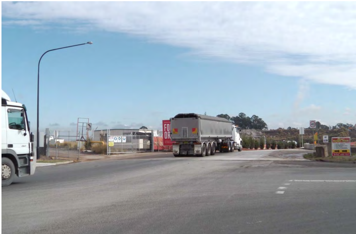
Photograph 2.1 Site access traffic using the intersection at Kangaroo Avenue/Honeycomb Drive
