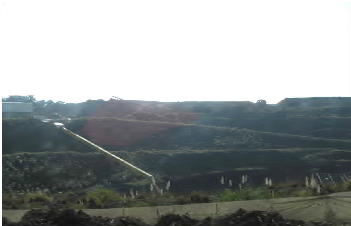
Photograph 2.16 View into the quarry showing chute for the disposal of special waste
