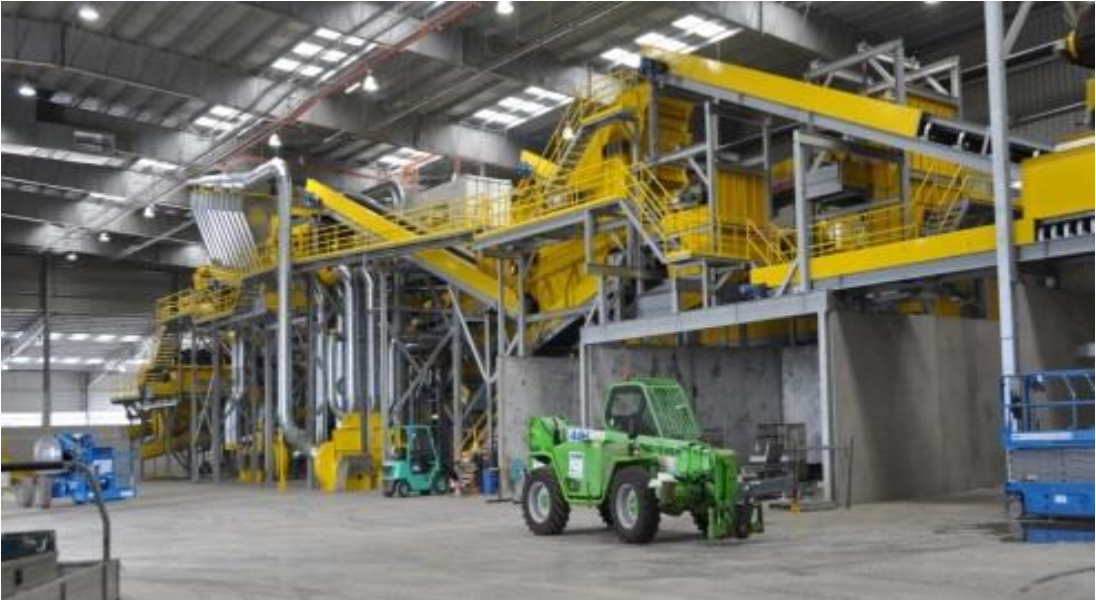
FIGURE 4 – VIEW OF PLANT INSIDE THE MPC (FROM THE NORTHERN END)
