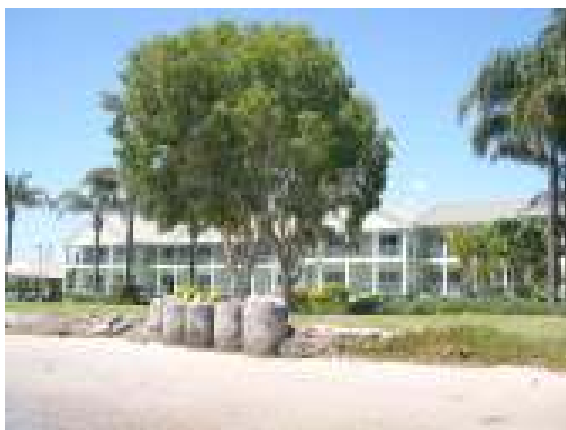
Figure 9: Moby Dick Hotel to the south of the site
