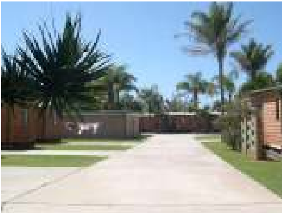
Figure 4: Cabins and concrete vehicle access ways
