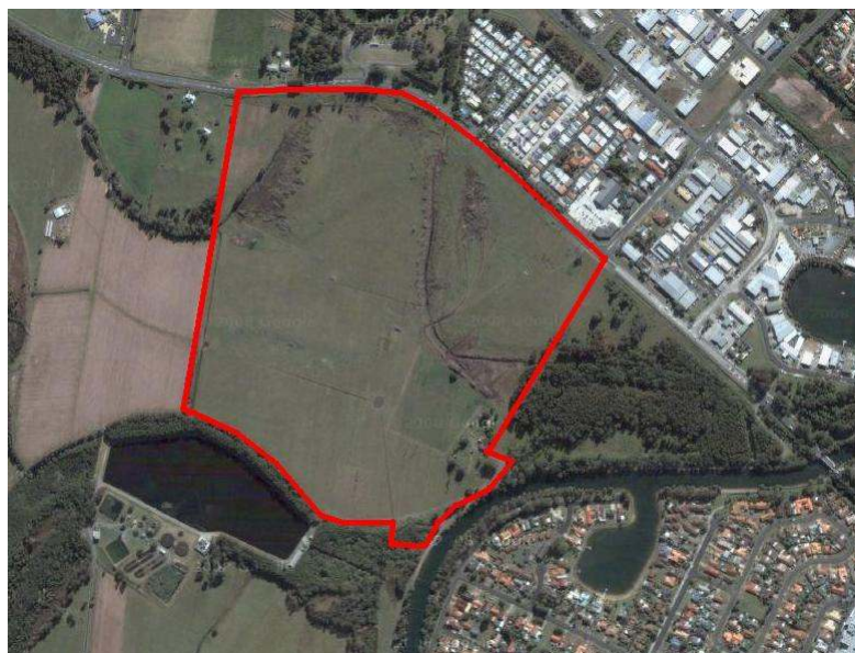
Plate 1 - Aerial photograph of the site prior to commencement of bulk earth works in accordance with development consent DA 2002/566.
