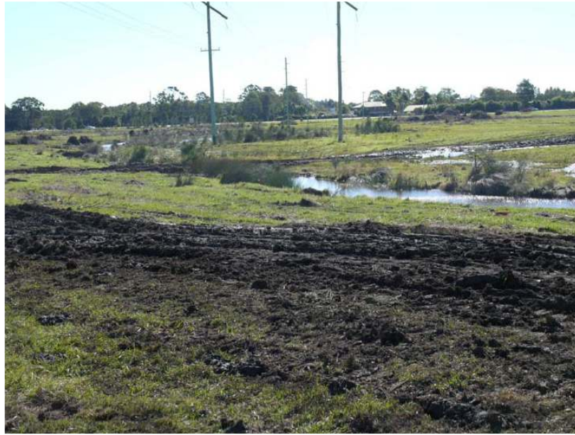
Plate 4 – View west showing the site post clearing of site's watercourse (Everick Heritage Consultants Pty Ltd 2007).
