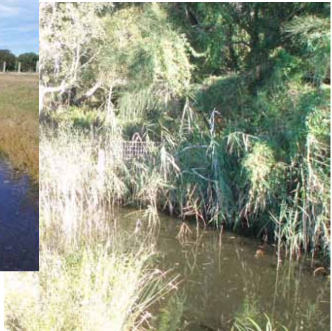
Plate 4. Existing drainage path entering Lot 1 DP1074242 south-western corner
