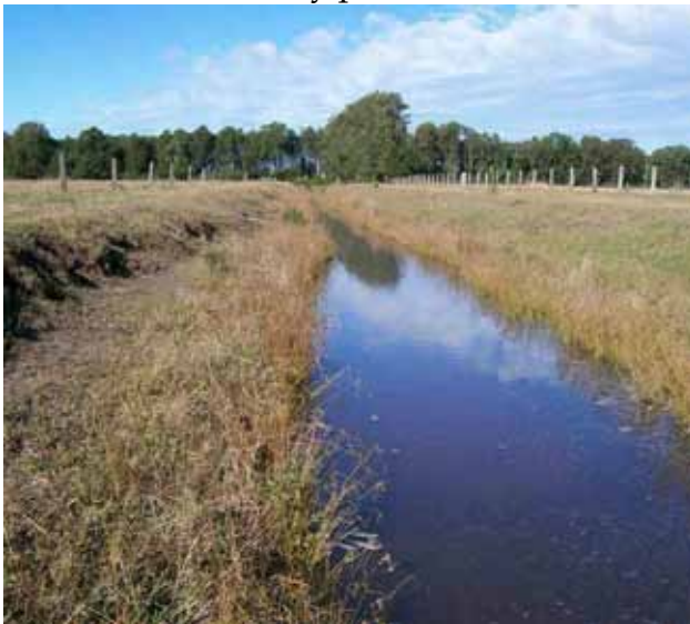
Plate 3. Existing drainage line running parallel Lot 2 DP1074242 western boundary
