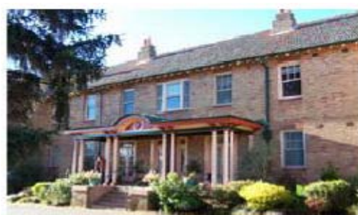
Photo 4 Gosling Creek Guest House
