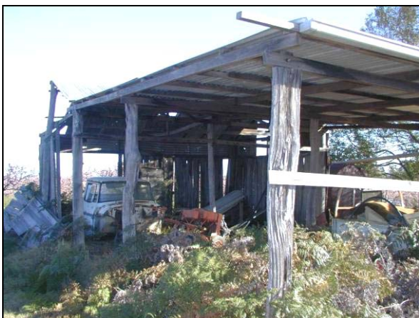
Plate 3. View of shed looking south
