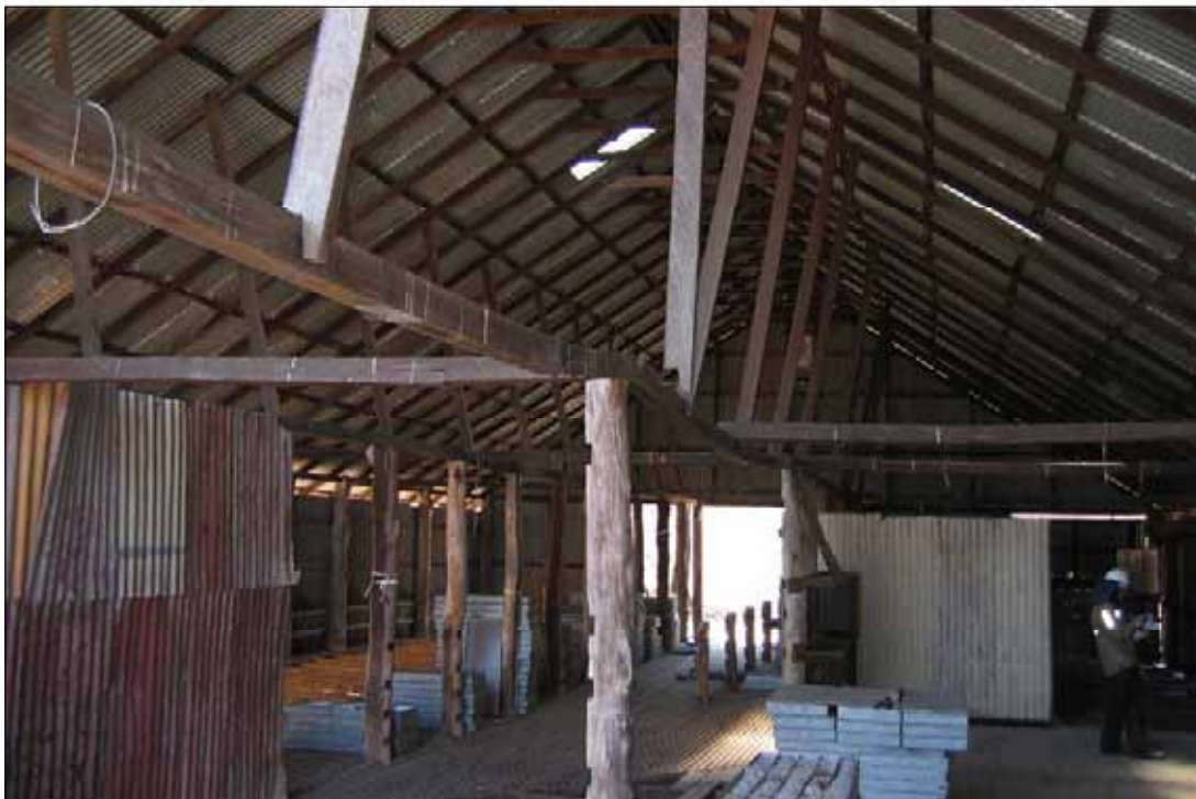
PLATE 14 Interior of Shearing Shed, Belmont Homestead
