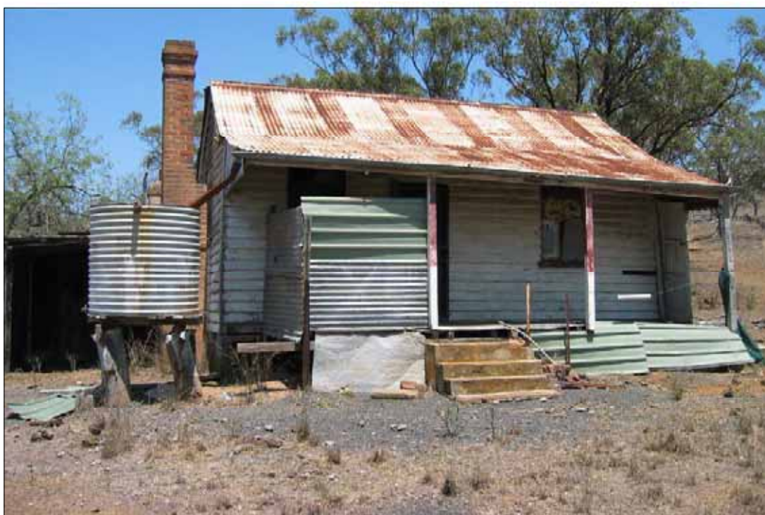
PLATE 8 Facing SW, overview of Mills Cottage
