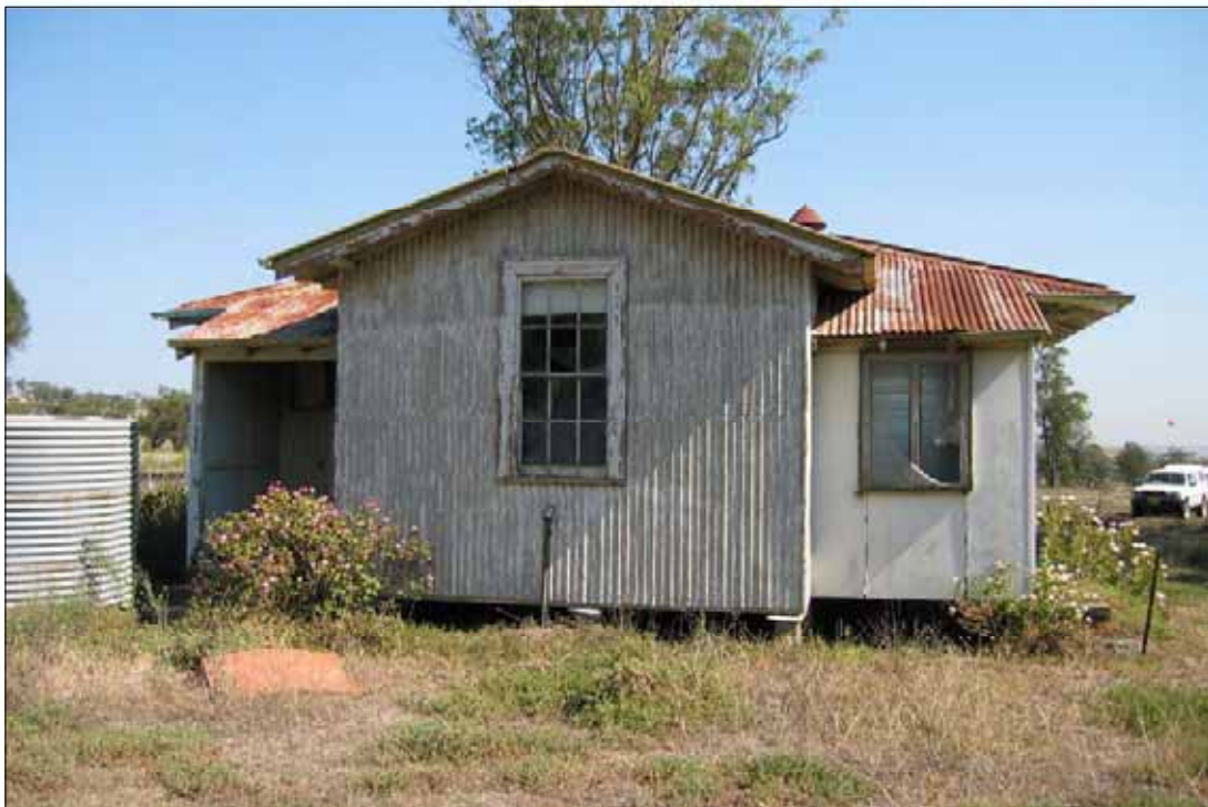
PLATE 4 Facing NE, Hospital Building
